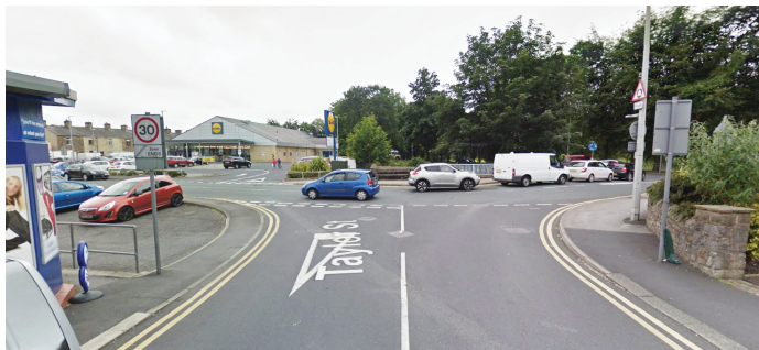
View showing of site from Taylor Street
