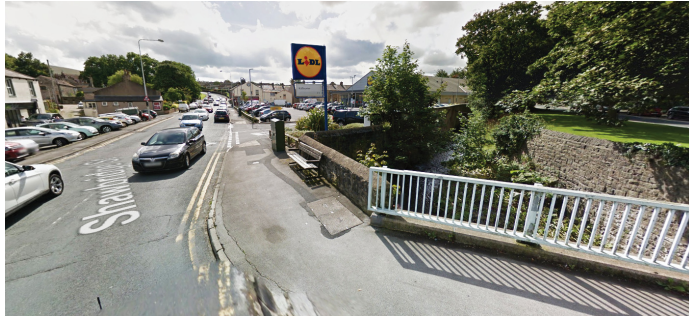
View showing the primary access to site
