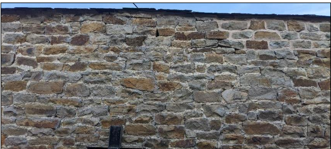
Plate 5. Open joints between masonry on northeast elevation of stone outbuilding
