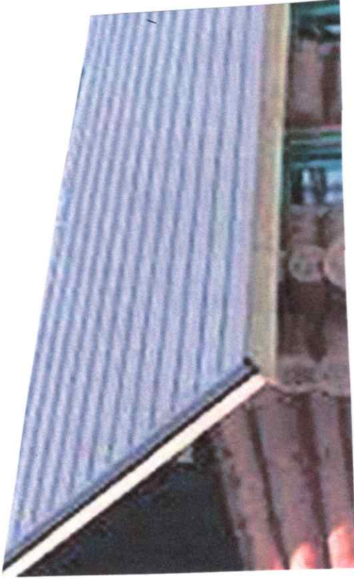
Log Cabin Roofs – metrotile lightweight roof shingles in DARK GREY , dark grey fascias and rainwater goods
