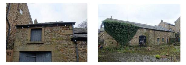
A detached two storey stone built barn is present to the west of the former public house. While the building is generally well pointed, gaps were present on gable ends, on external walls and at the eaves. Some lifted slates were recorded and gaps were present along ridge tiles.
