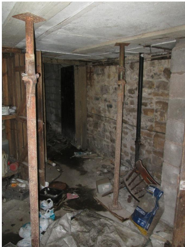
Photo 20 – Propped roof to covered yard
