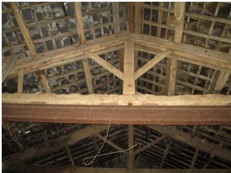
Photo 24 – Barn roof structure
