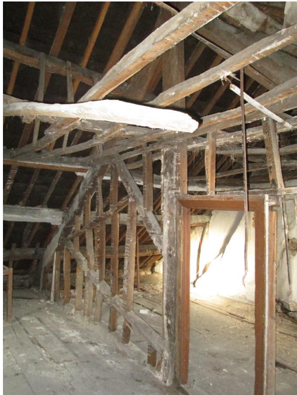
Photo 9 – Truss strut removed to form door opening
