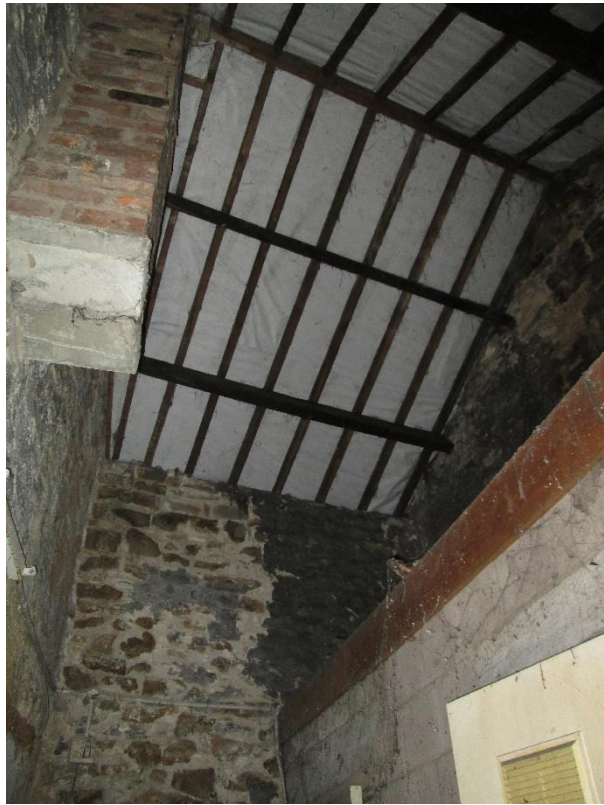
Photo 21 – New roof to front right-hand storeroom
