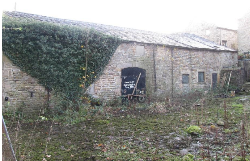
Photo 4 – View of rear of barn
