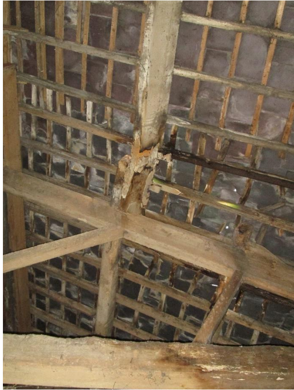
Photo 25 – Fractured purlin
