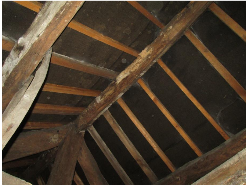
Photo 5 – Underside of roof, showing new rafters and felt
