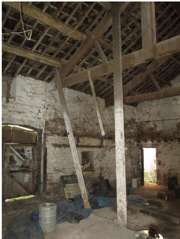
Photo 26 – Timber uprights fixed to truss
