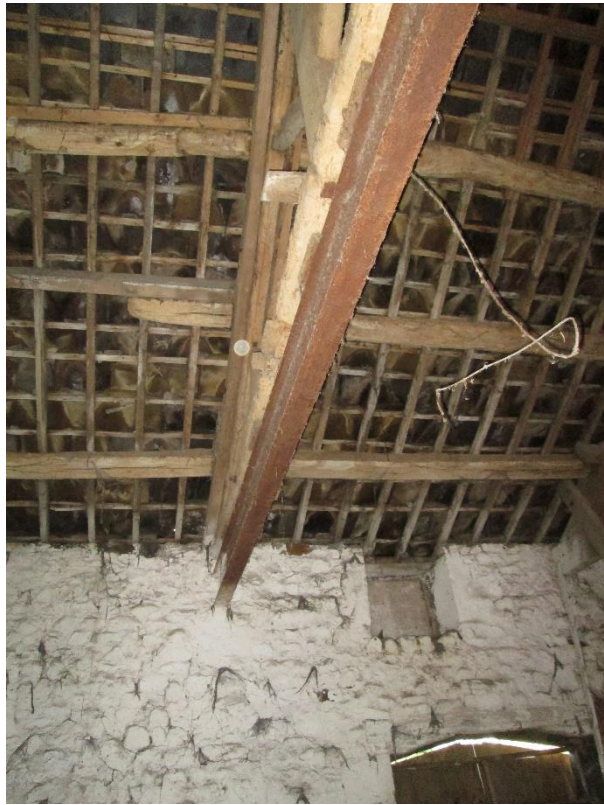
Photo 27 – Steel beam below third truss
