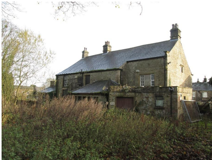
Photo 2 – View of rear of hotel
