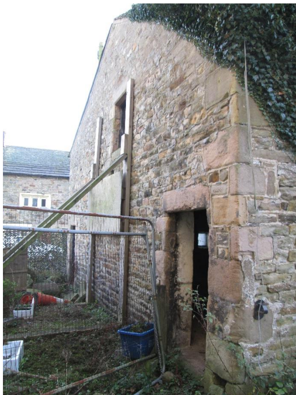
Photo 32 – Propped gable wall
