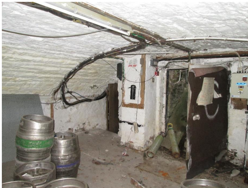
Photo 22 – General view of cellar
