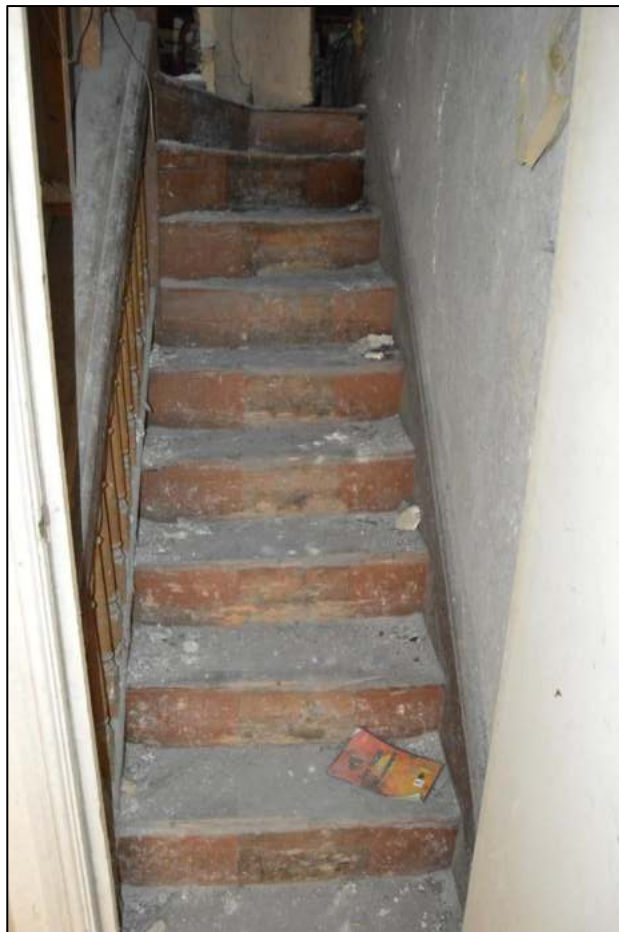
PL62: View of attic staircase.
