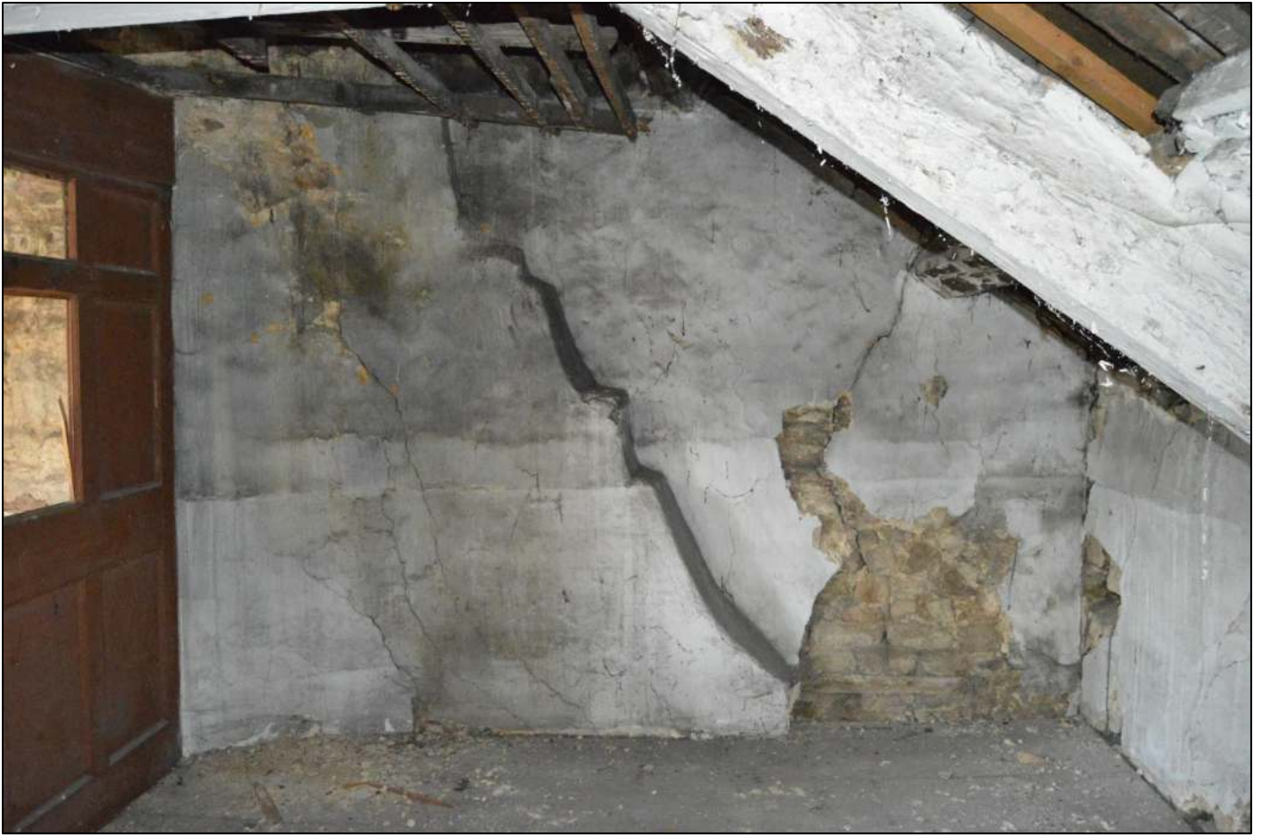
PL71: View south west within the south unit of the attic.
