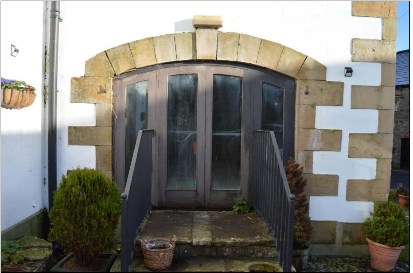
PL07: View of the former coach entrance to the south west elevation of the 19th century coach house addition.
