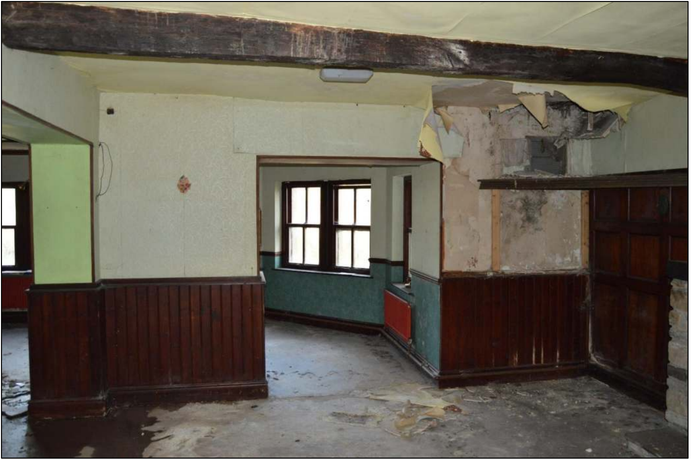
PL29: View north west within the ground floor north unit.
