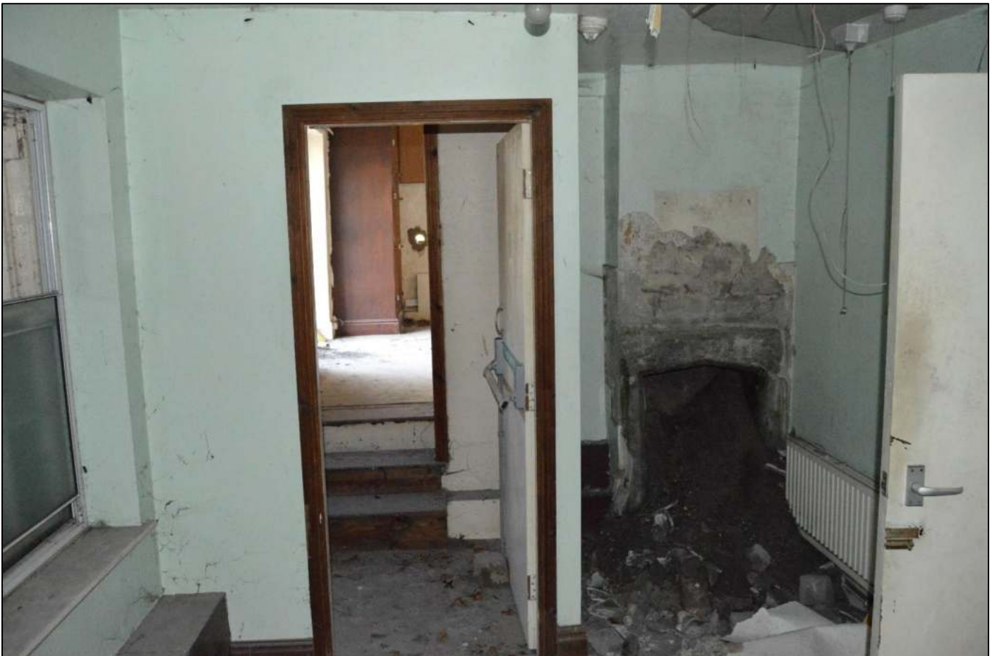
PL42: View north east within the first-floor north unit.
