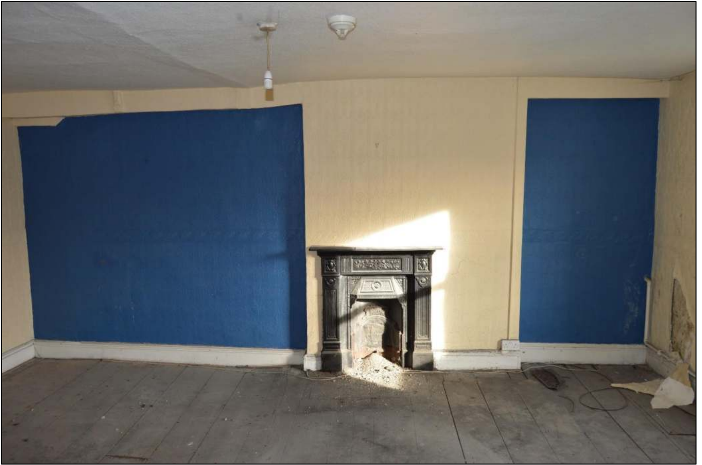
PL55: View north east within the first-floor east unit.
