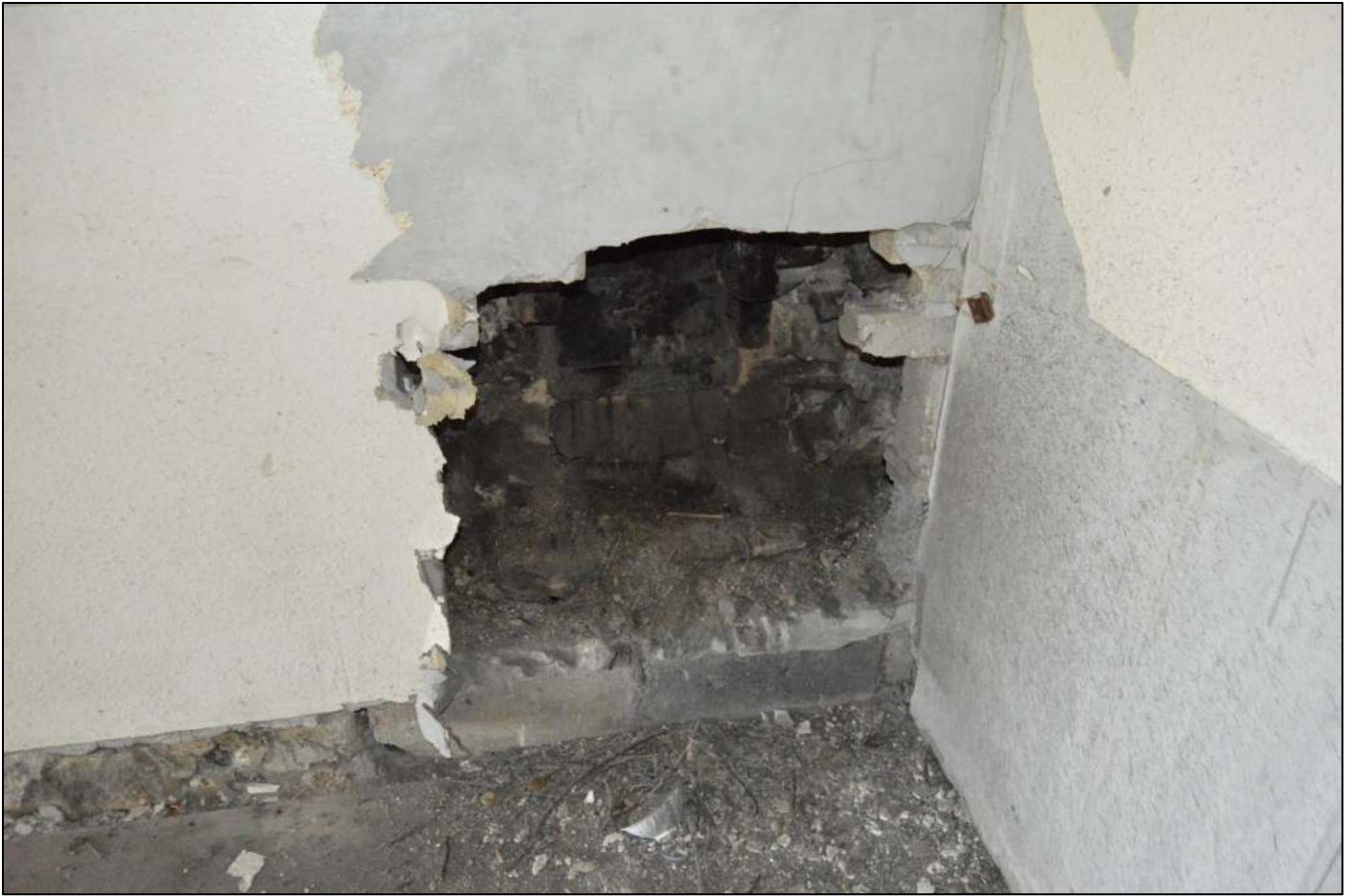
PL41: View of former fireplace opening to the chimney breast to the rear first floor unit of the coach house addition.
