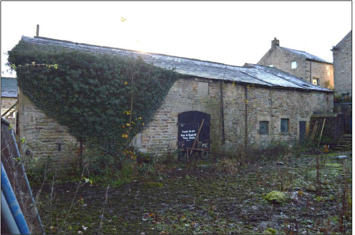
PL79: View of the barn from the north.
