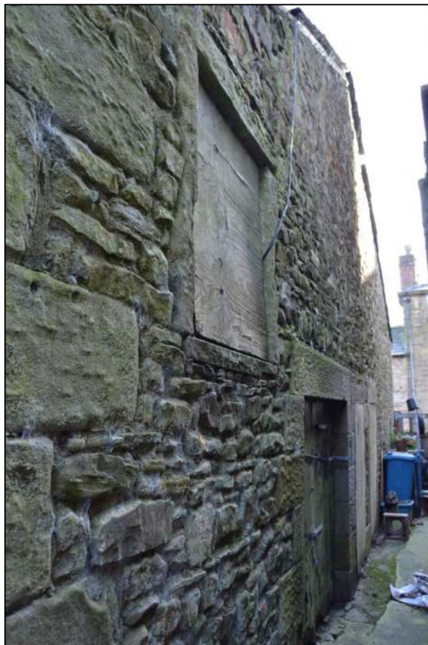
PL78: View of the south west gable from the north.
