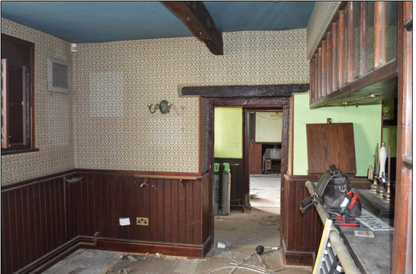
PL21: View south west within the ground floor east unit.
