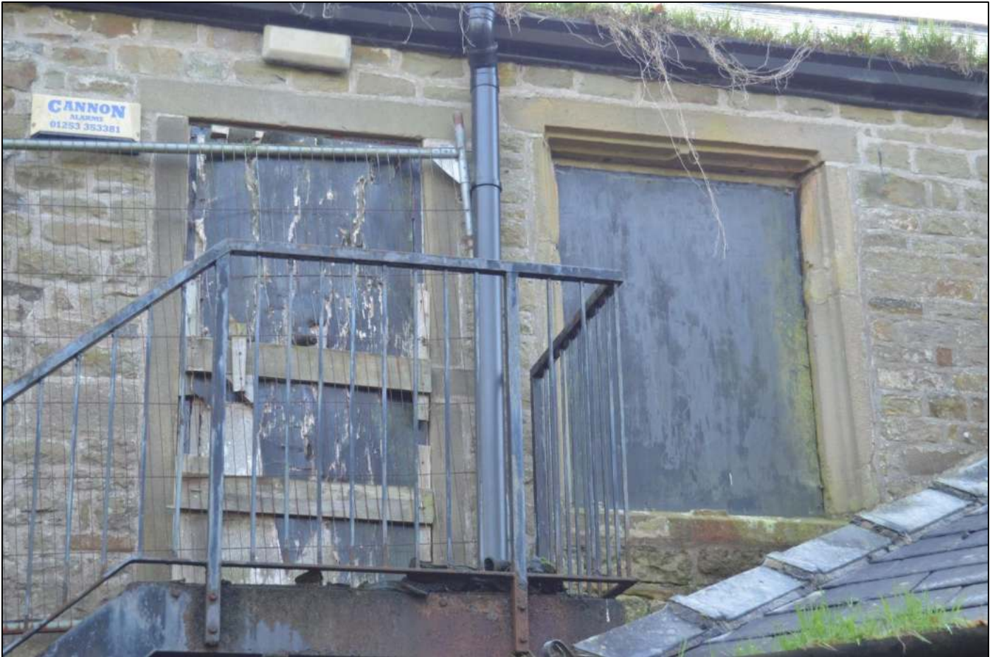
PL13: View of the inserted first floor doorway and the re-used 17 th century former cross window (mullion and transom missing).
