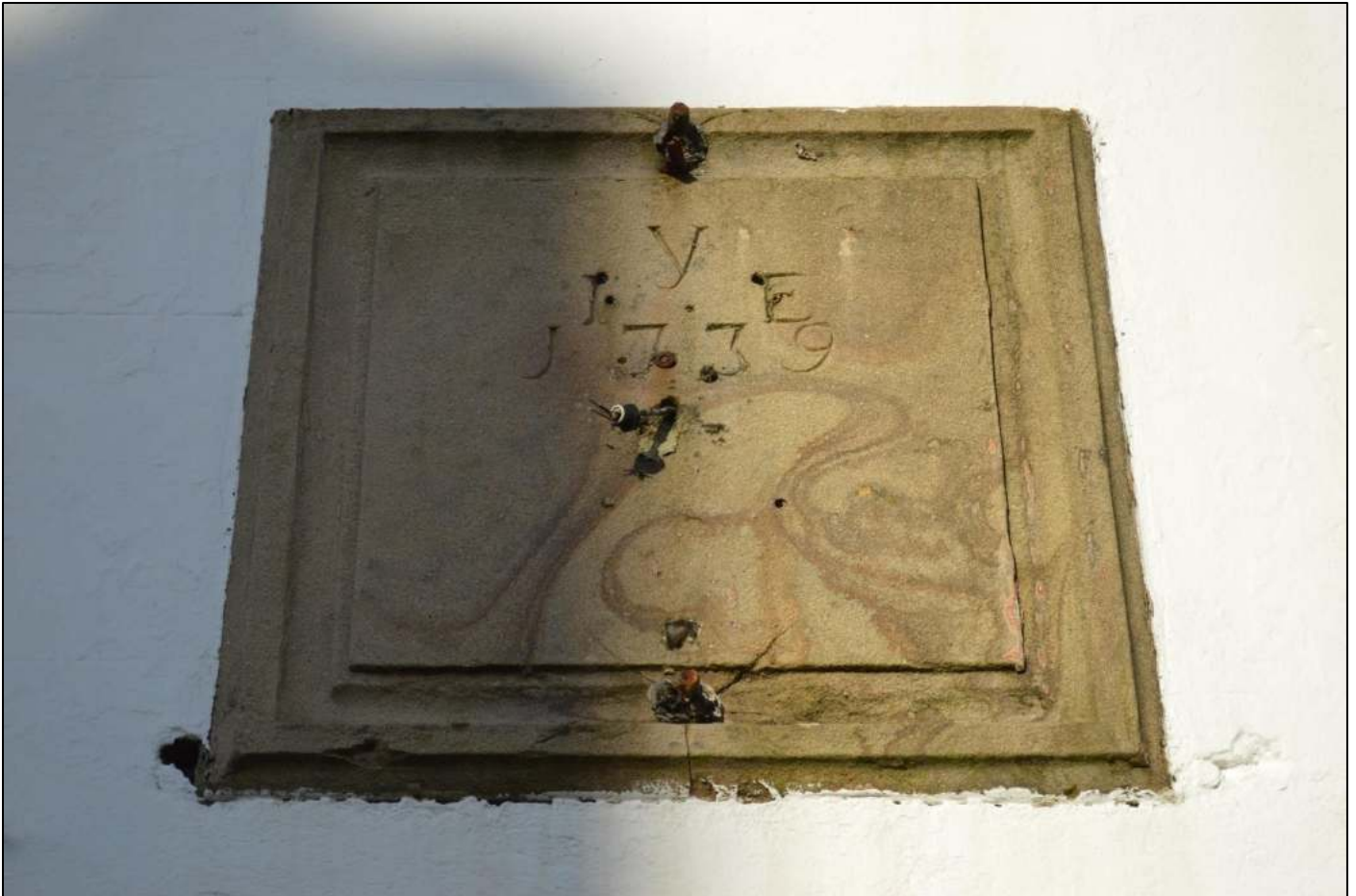
PL03: View of the date stone to the front South East facing elevation of the Talbot Hotel.
