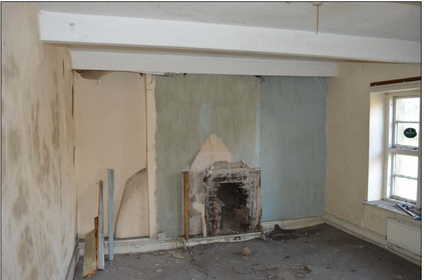
PL60: View south west within the first-floor west unit.
