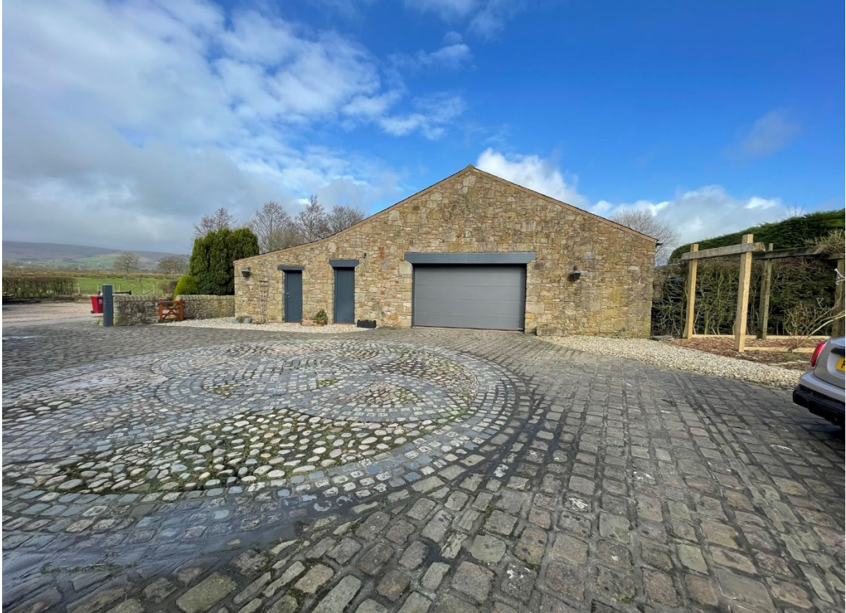
View of the garage from the driveway of Pale Farm Barn.
