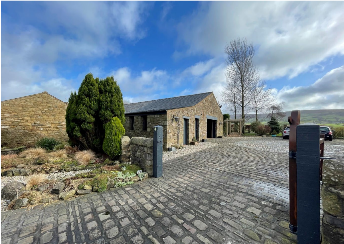
View from the access gates at Pale Farm Barn.
