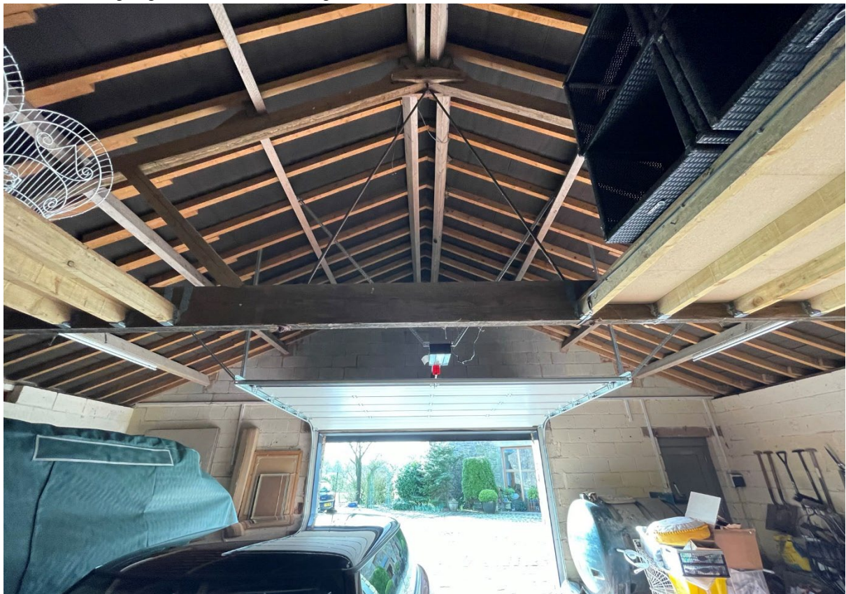
Internal view of garage.
