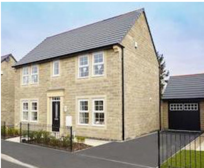
Fig 2.4. Example of railings around enclosure in Clitheroe
