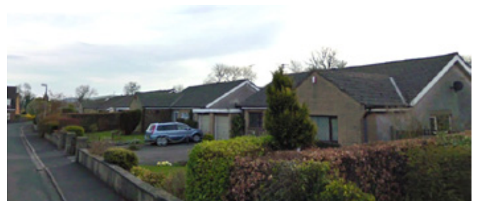
Fig 4.3. View of bungalows on Gills Croft
