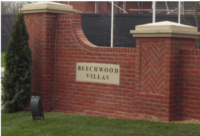
Fig 3.2. Sign incorporated into wall
