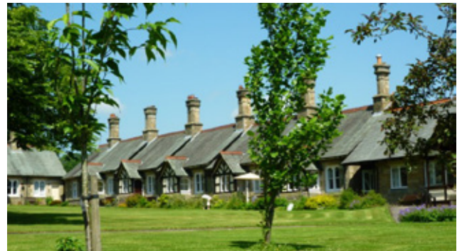
Fig 4.30. Single storey Alms Houses formerly Waddington Hospital
