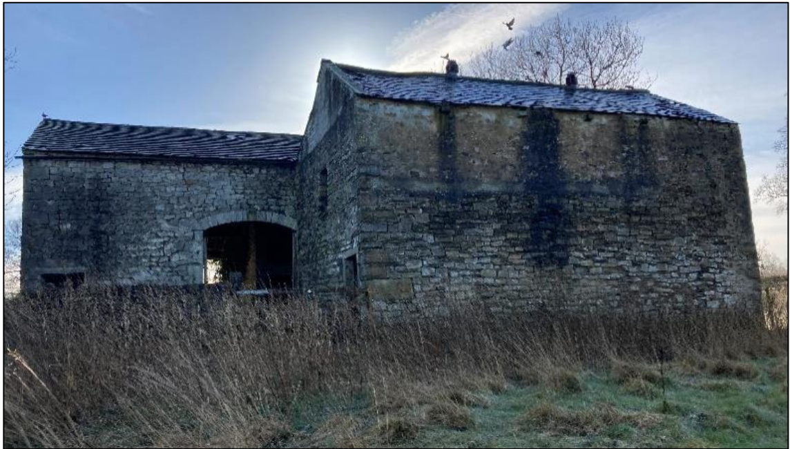
Plate 11. West-Facing Elevation of Little Moor Farm
