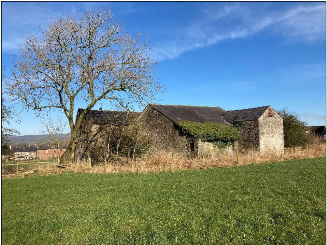
Plate 10. Northwest Elevation Facing Towards Little Moor Farm
