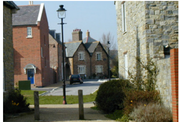
Fig 3.3. Example of feature street lighting
