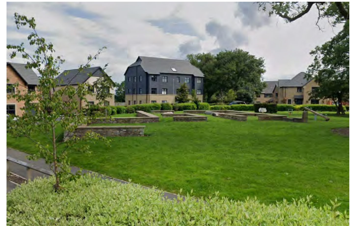
Example image of converted Bothy in Higher Standen Phase 1
