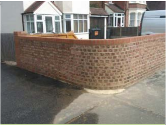
1800mm Curved Brick wall
