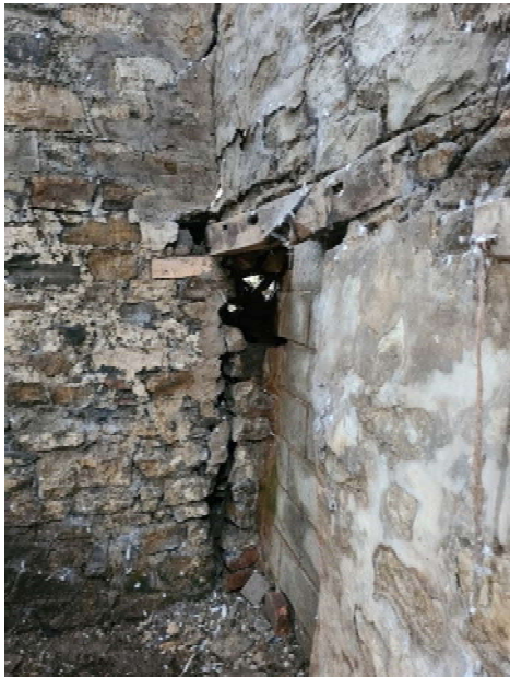
Image 4 showing significant and severe separation of wall junction, partly due to blockwork rigid infill Image 5 showing blockwork infill and resultant severe vertical cracking
