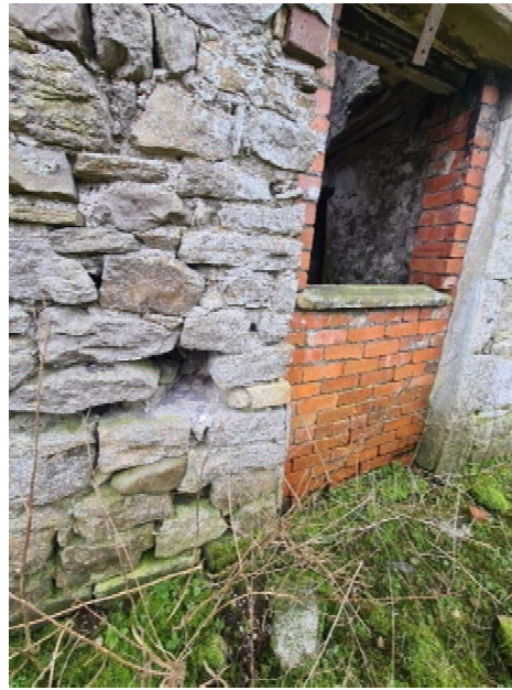
Image 2 showing collapse of wall at apex and evidence of cement based mortar repair in stonework and associated vertical cracking at the interface of the two different mortar types. Image 3 indicating non sympathetic masonry infill and rigid panel
