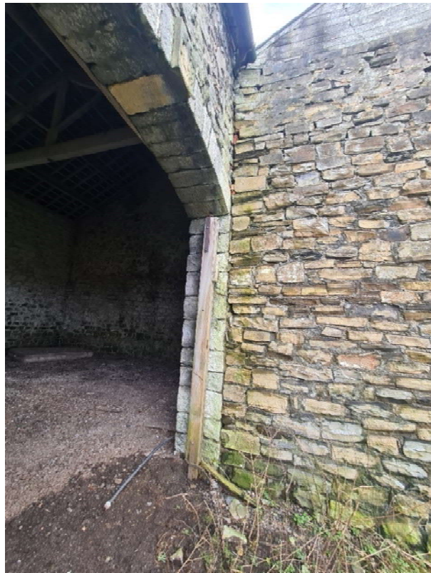
E9 - Arch and vouzsoirs in good order. Clear vertical break to west
