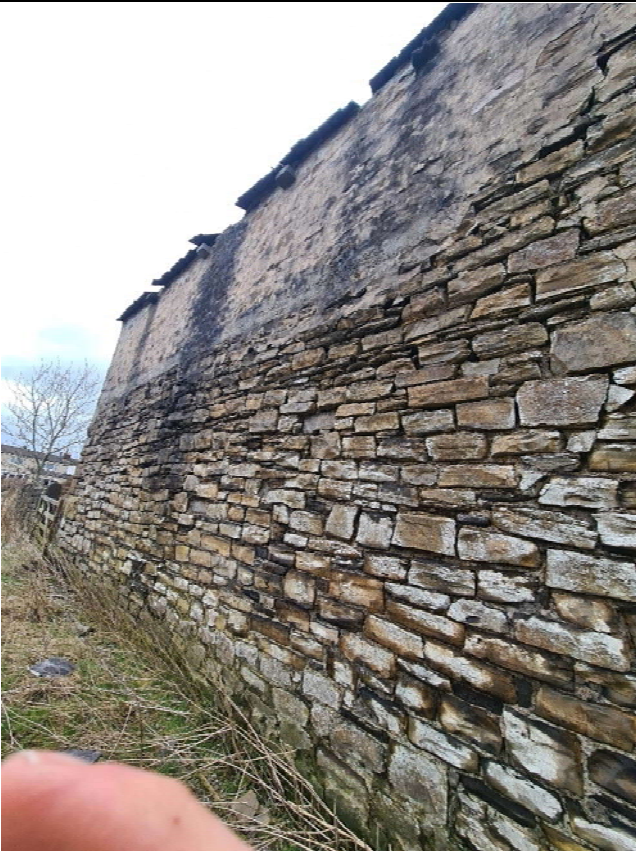
E5- Cementitious render and water staining
