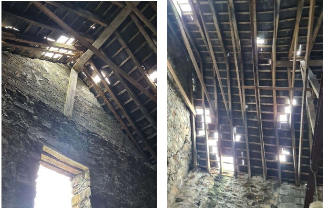
Image 10 showing rebuilt blockwork pediment and plank upright supporting ridge plank. Image 11 showing lack of ridge support and high collar ties that are not as per original construction and allowing lateral thrust on the walls that never existed in the original construction arrangement.
