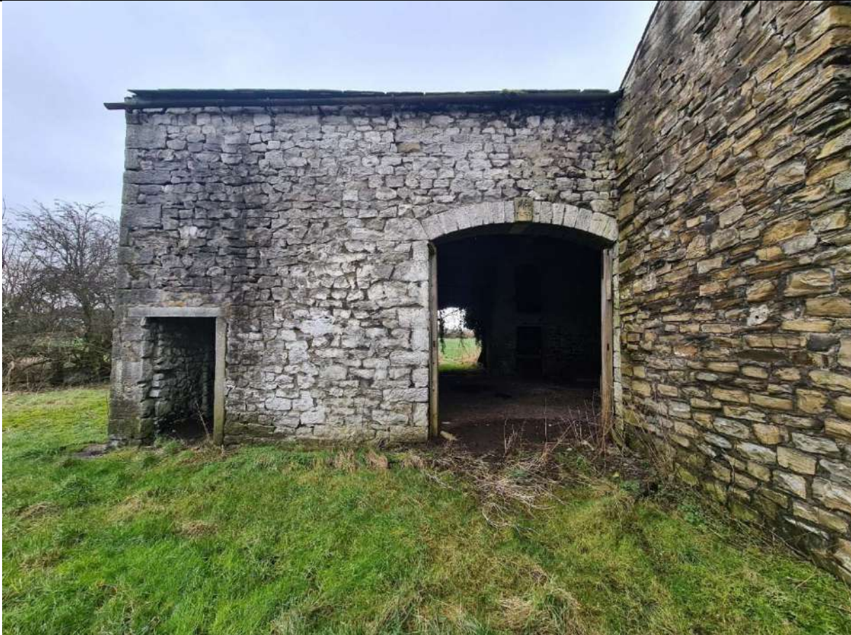
E7 - Water staining, repointing required - generally in good order
