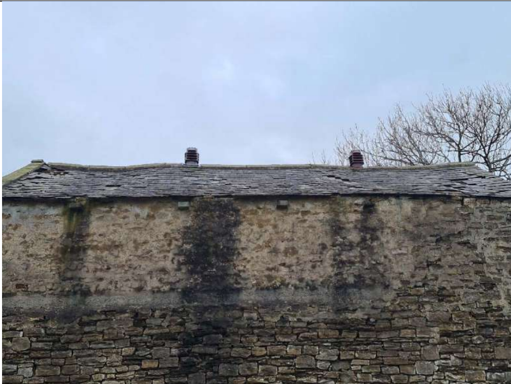
E2- Undulating roof – cementitious render and repointing evident
