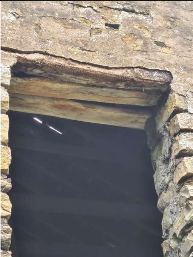
N6 - Timber lintels weather damage and insect attack observed
