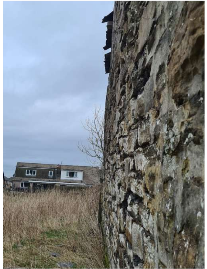
E4- Wall out of plumb and cementitious repointing
