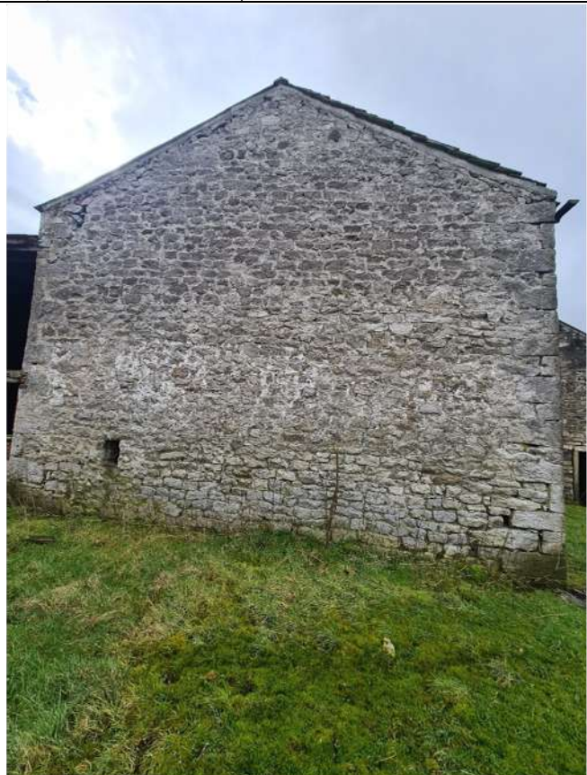
N7 - Diagonal cracking in left hand corner
