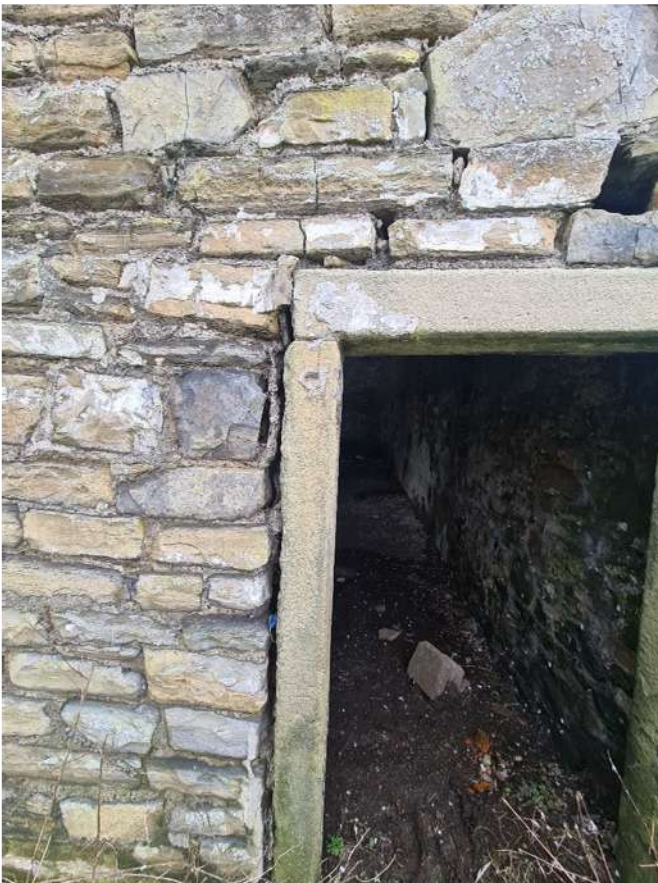
N4- Separation of stone door frame
