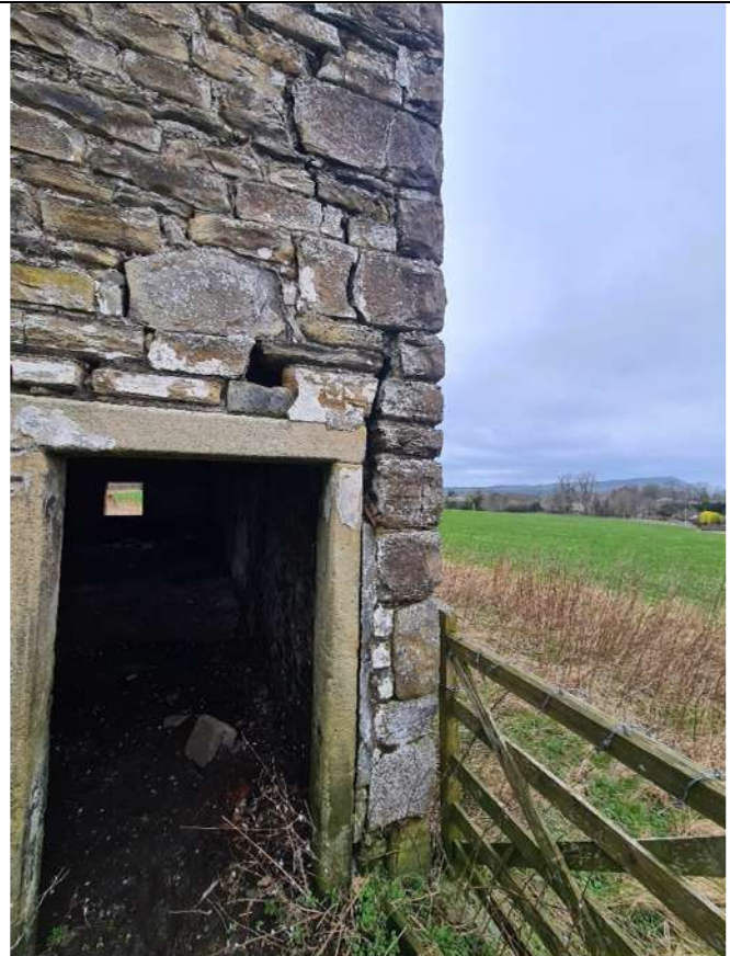
N3- Separation of east elevation wall evident in vertical cracking
