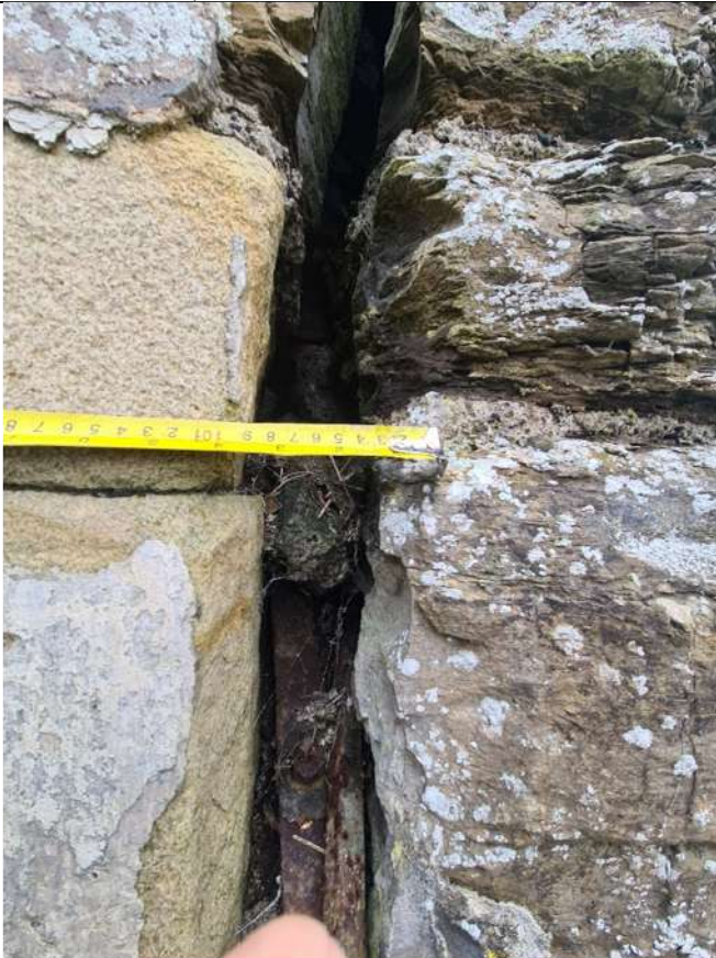
N2 – 90mm separation from stone door frame – corroded metal
