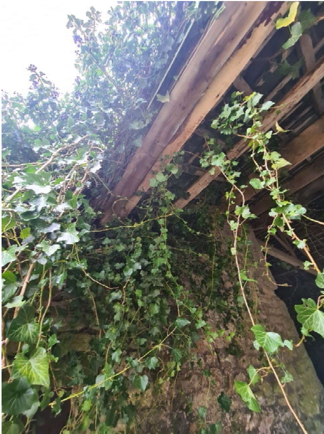
W6 - Ivy holding moisture near timber elements
