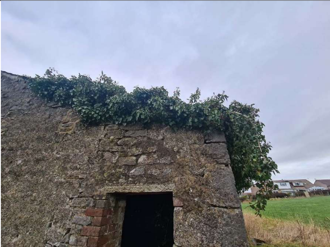
S2 – Ivy growth, cementitious render, masonry infills observed
