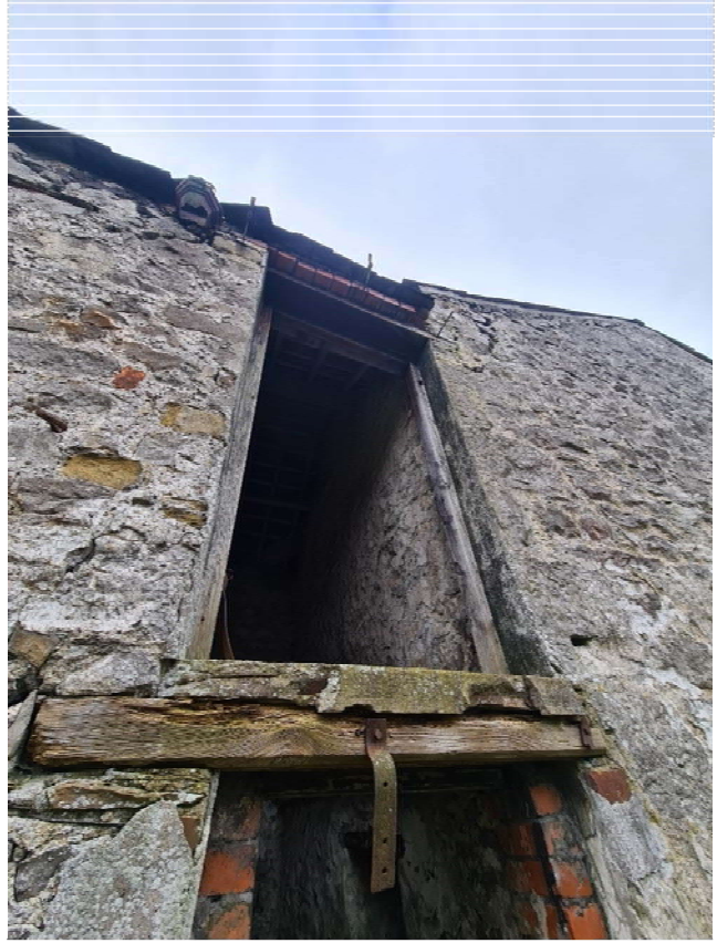
N13 – Wall distorted around masonry infill, weather damaged lintel
