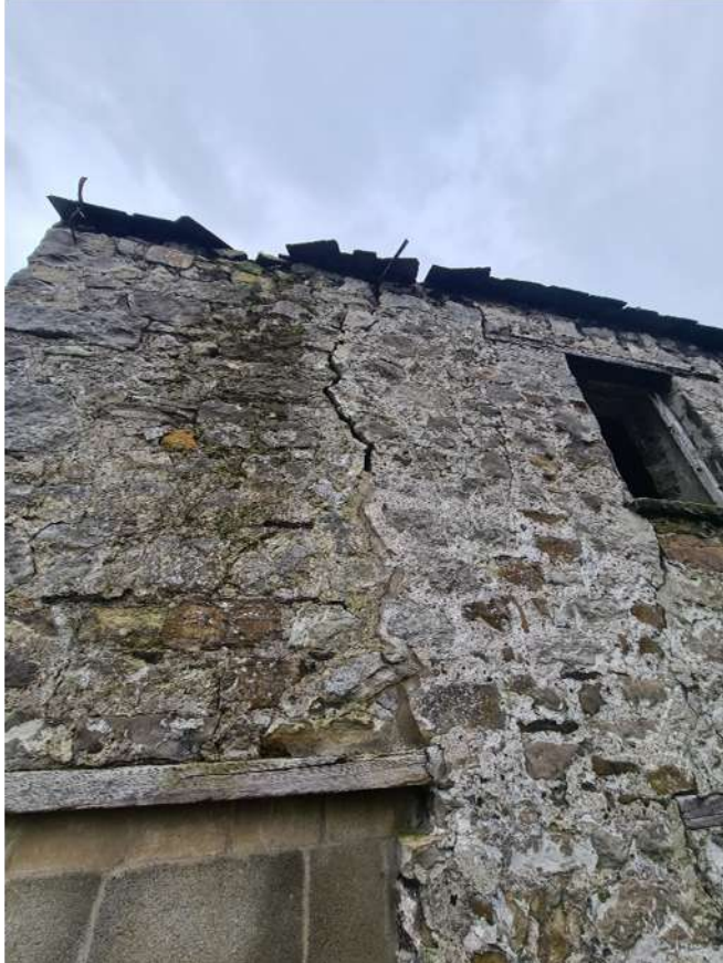
N10 – Severe vertical crack at area of rigidity below (in-fill)
