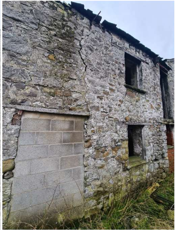
N9 – Block infill and severe vertical cracking along the reveal line
