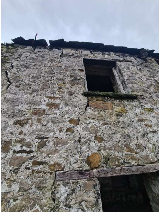
N14 – General vertical cracking at reveals of doors and windows
