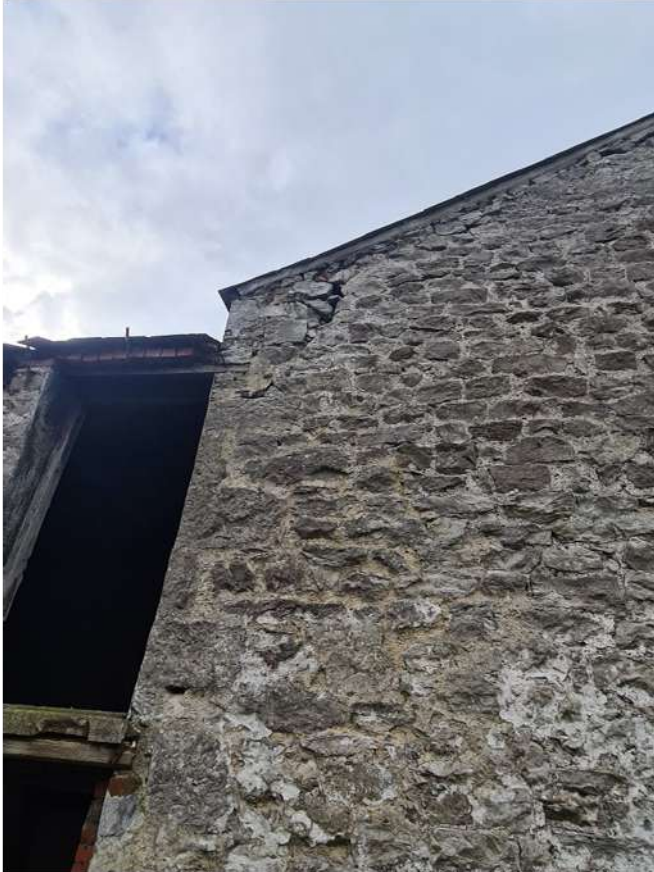
N8 – Diagonal cracking at corner
