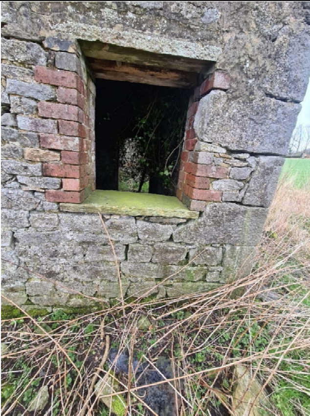
S4 - Poorly maintained (re-pointing required), masonry in-fill
