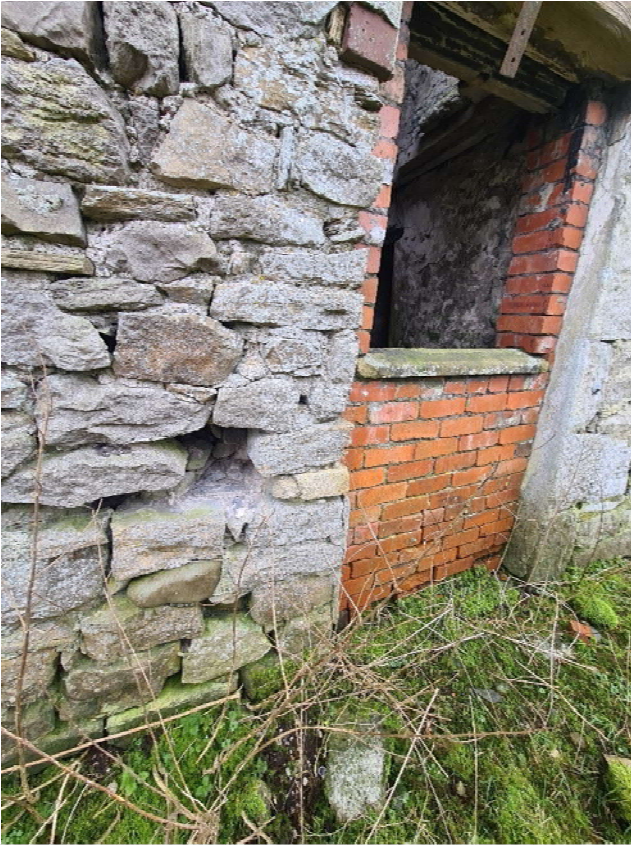
N12 – Masonry in-fill and poorly maintained mortar
