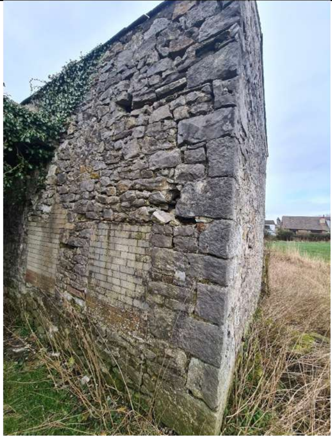
W4- masonry in-fills, poorly maintained façade repoint and stone infill
