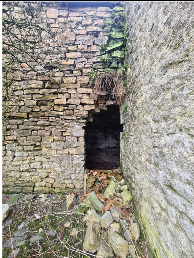
W9- Collapse of masonry in-fill and stone above, wall in poor condition, mortar joints eroded and bulging evident
