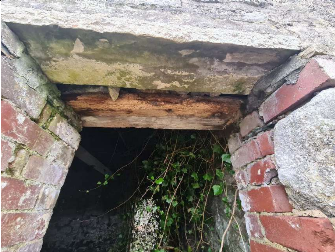
S3 - Water and insect attack on timber lintel, lintel timber flaking and soft
