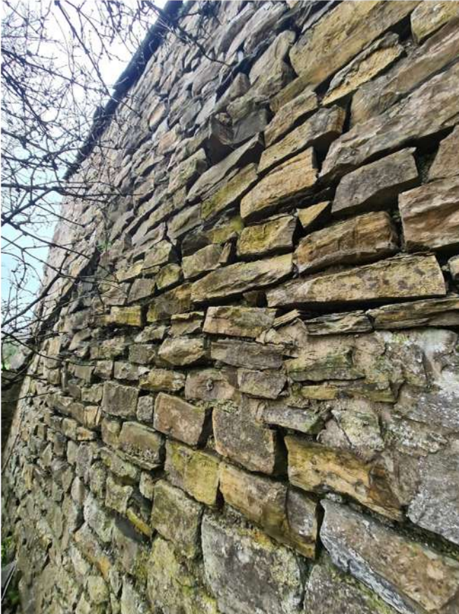
W10 – Mortar joints eroded, wall bowing and stone loose
