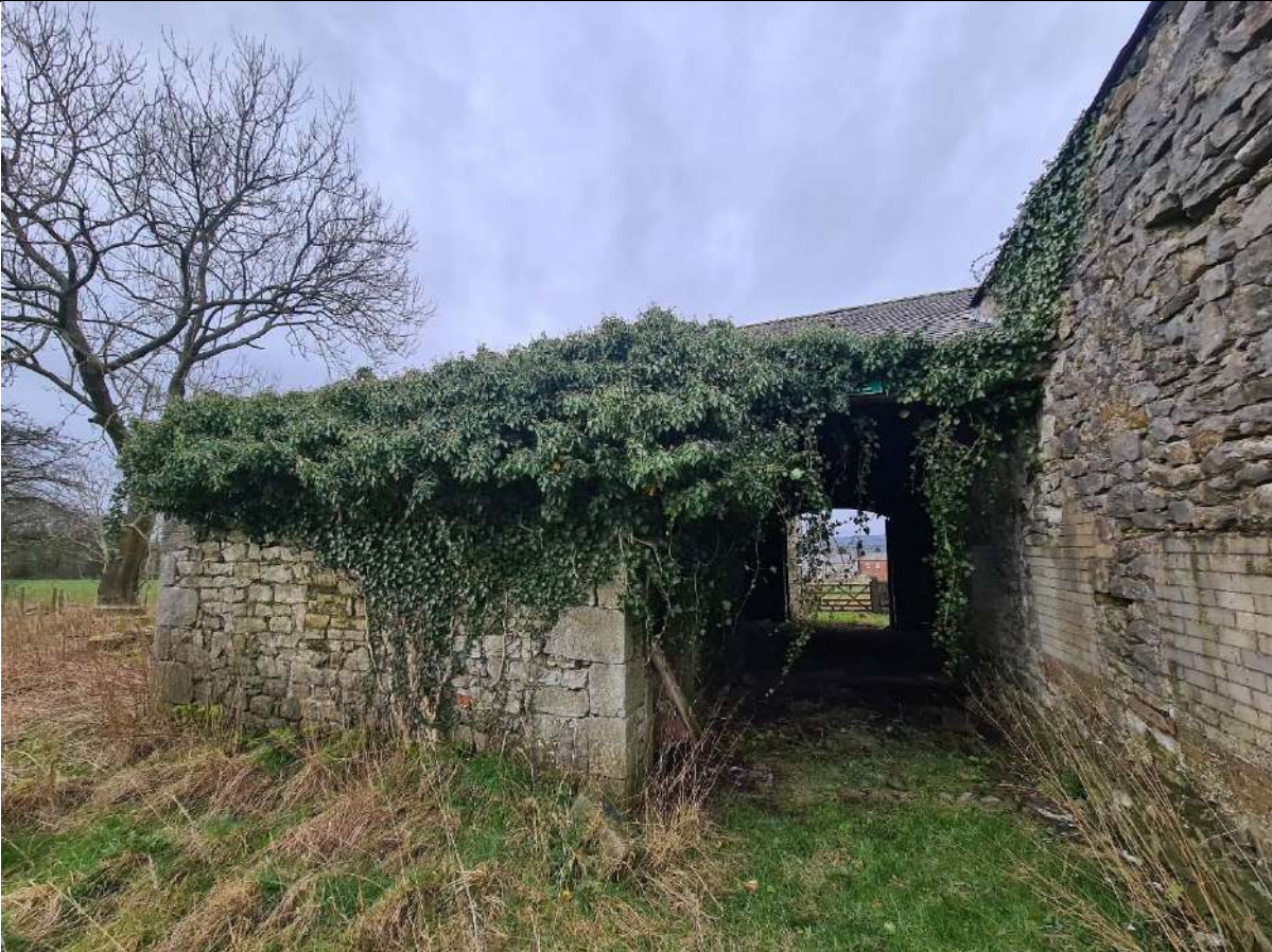
W5 - Ivy growth very severe on roof and south side of elevation
