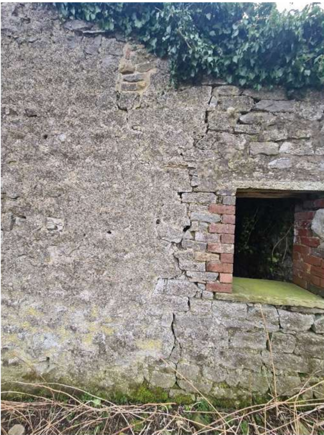
S6 – Vertical cracking at junction of cementitious render
