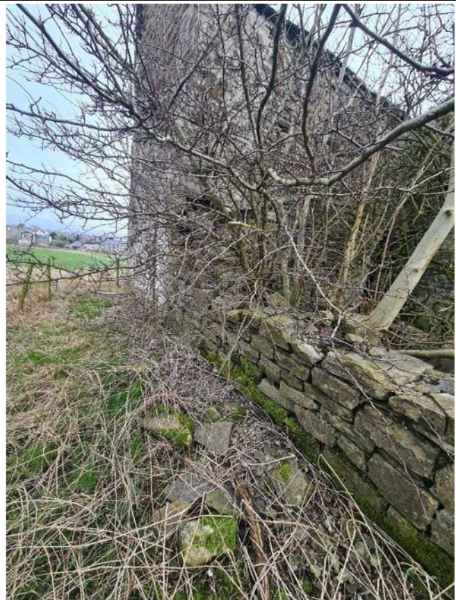
W13 – External wall fixed to elevation and rotating due to tree
