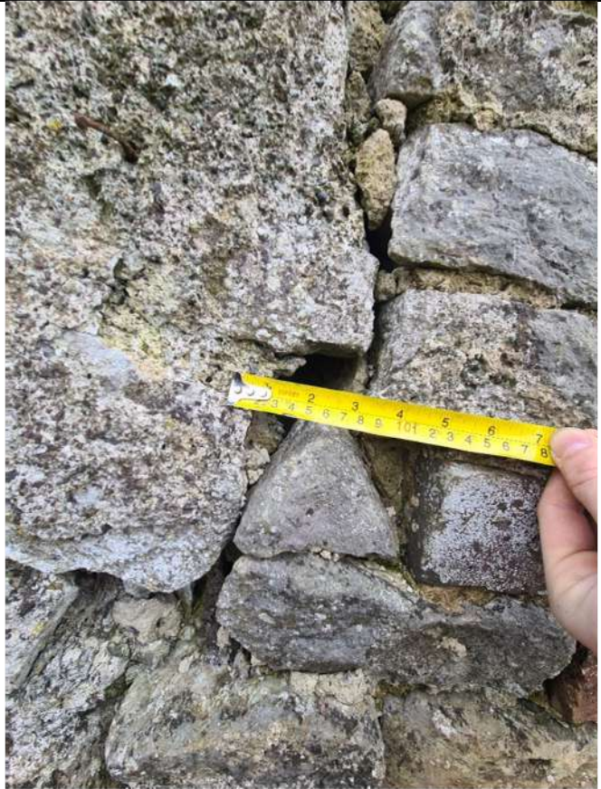
s7- Max crack width on S6 of 30mm
