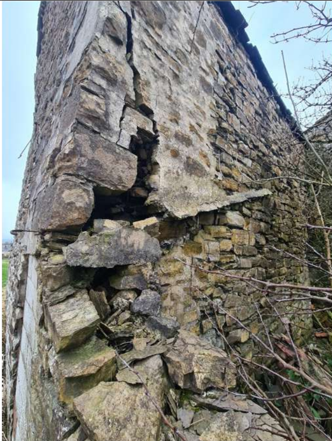
W12 – Severe crack and distortion of wall
