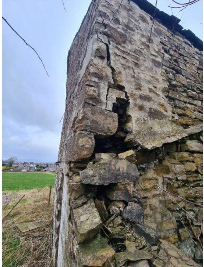
W11 – Cement repointing and infill, severe crack and separation
