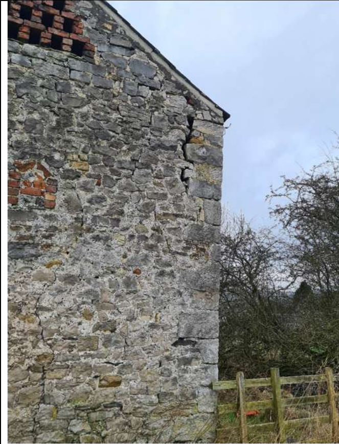
W3 - Cement mortar repointing and severe vertical crack at eaves
