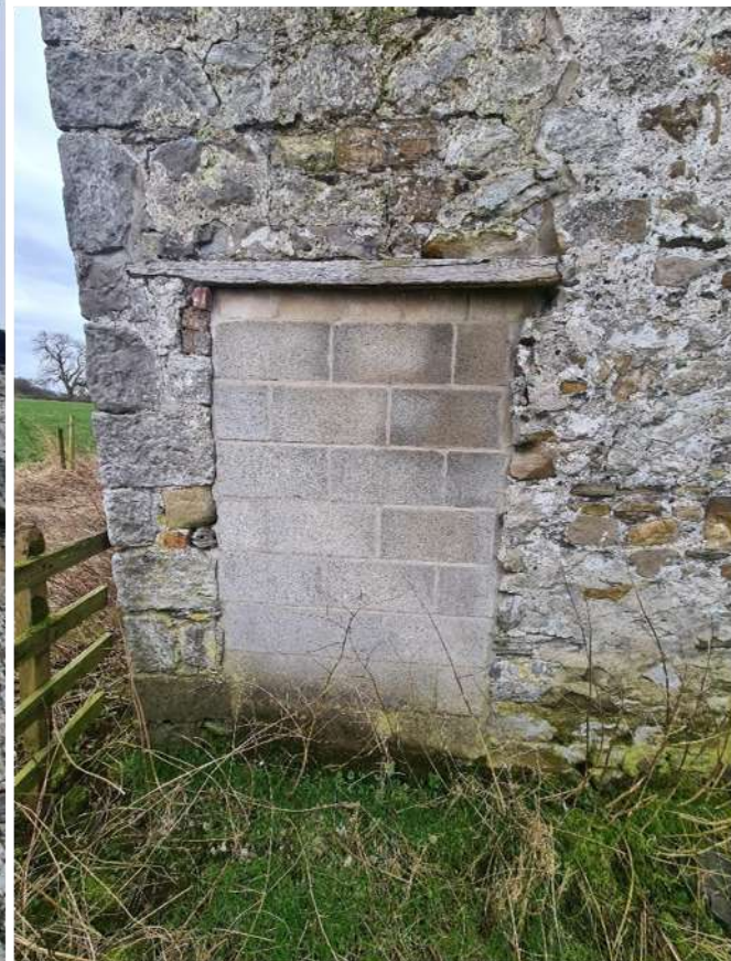
N11 – Blockwork in-fill in cement mortar
