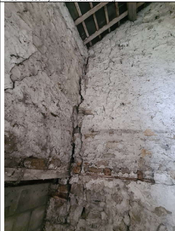
IN12 – Seperation of elevation walls
