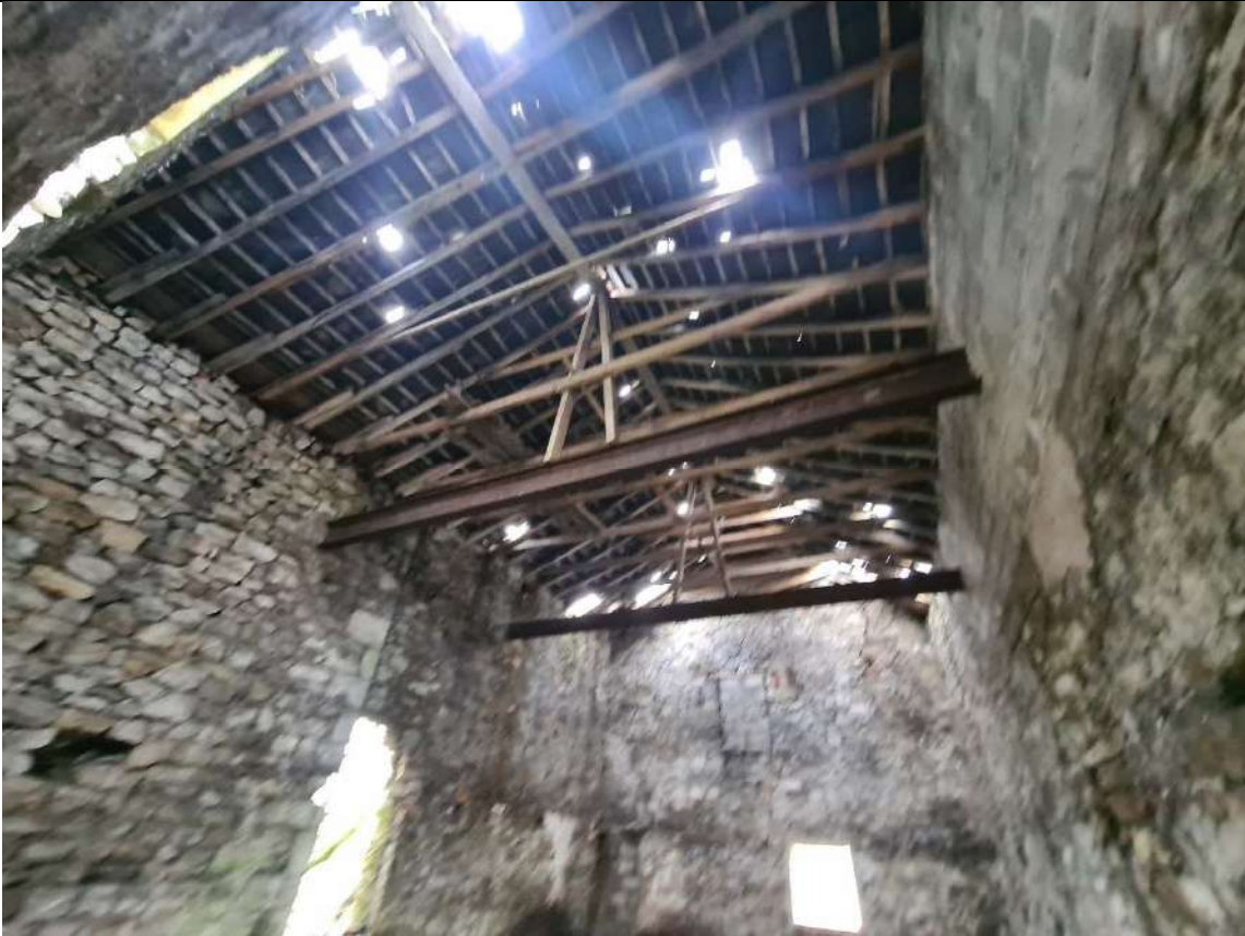
IN15 - Western section roof, steel UBs used to prop ridge in unorthodox fashion
