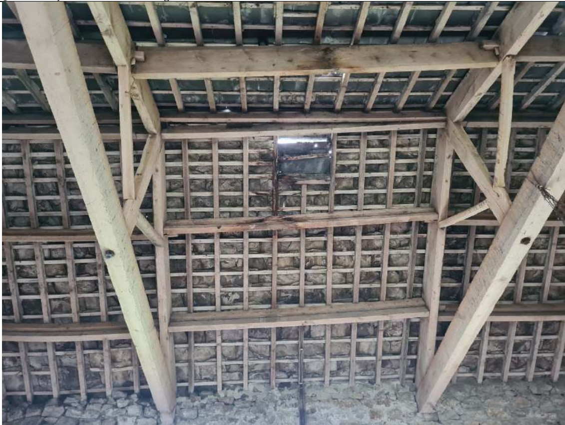
IN14 – Eastern section roof, some water ingress and staining noted
