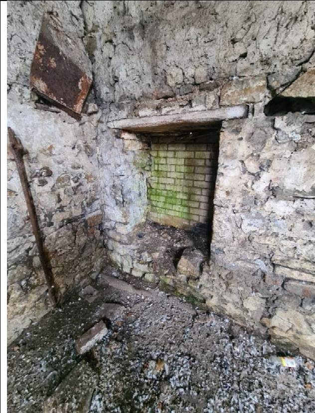
IN10 – Masonry in-fills, water staining
