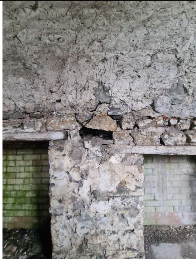
IN11 – Defelcting lintels and stone in-fill required
