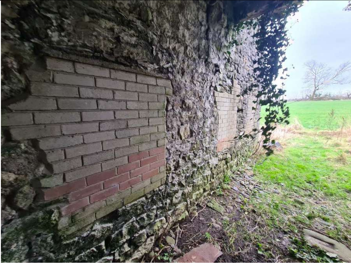
IN13 – Masonry in-fill – water staining at base
