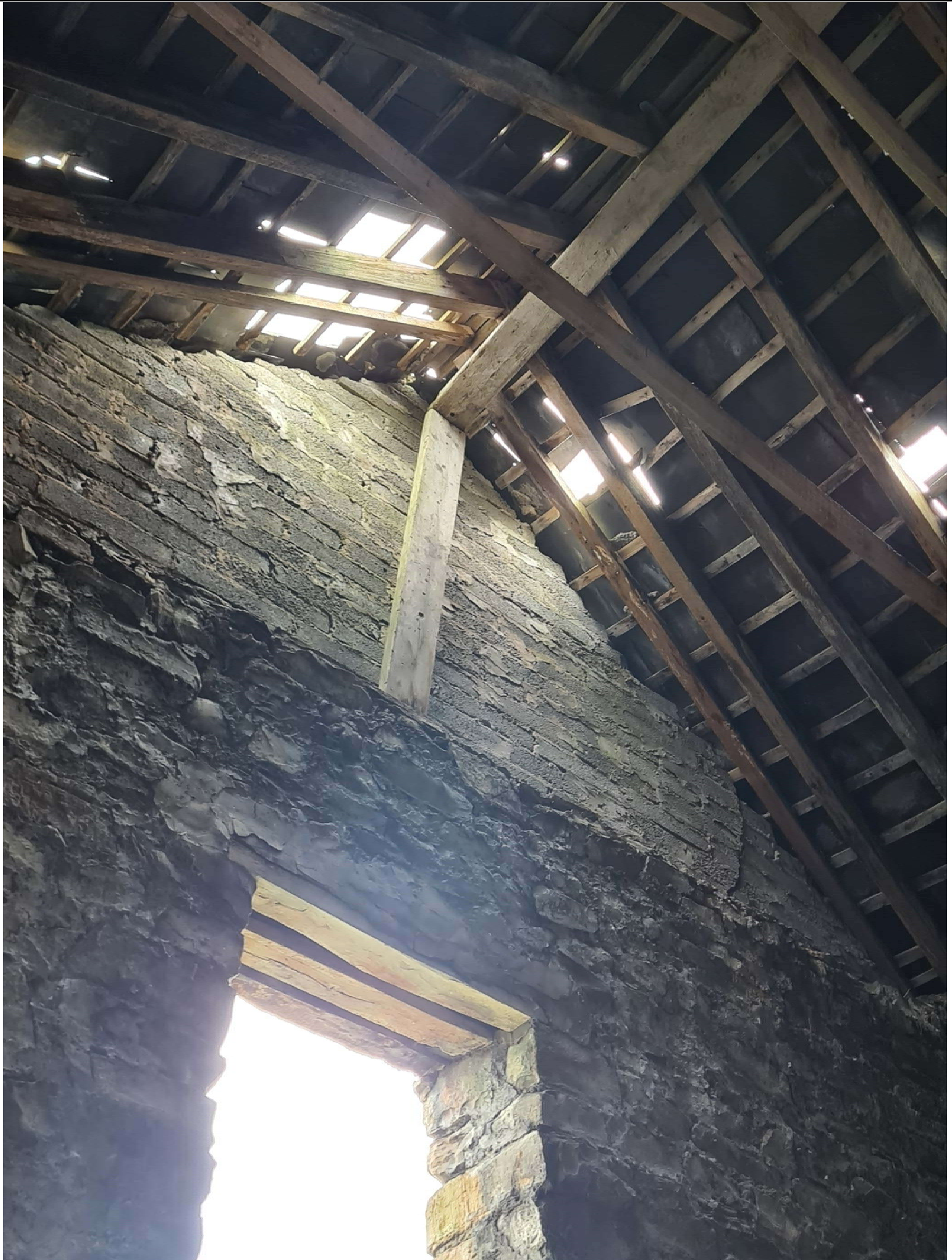
IN17 - Timber ridge support dangerous and anticipate collapse upon further degradation of planks
