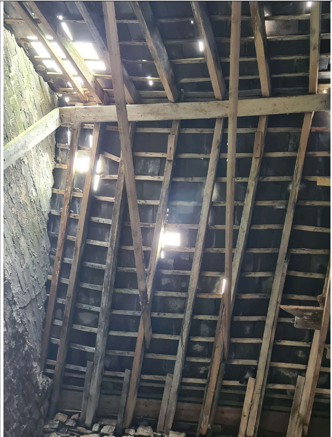
IN18 – Timber ridge support severely deflecting, and roof layout skewed in response to movement and lack of support – infrequent or nonexistent collar ties
