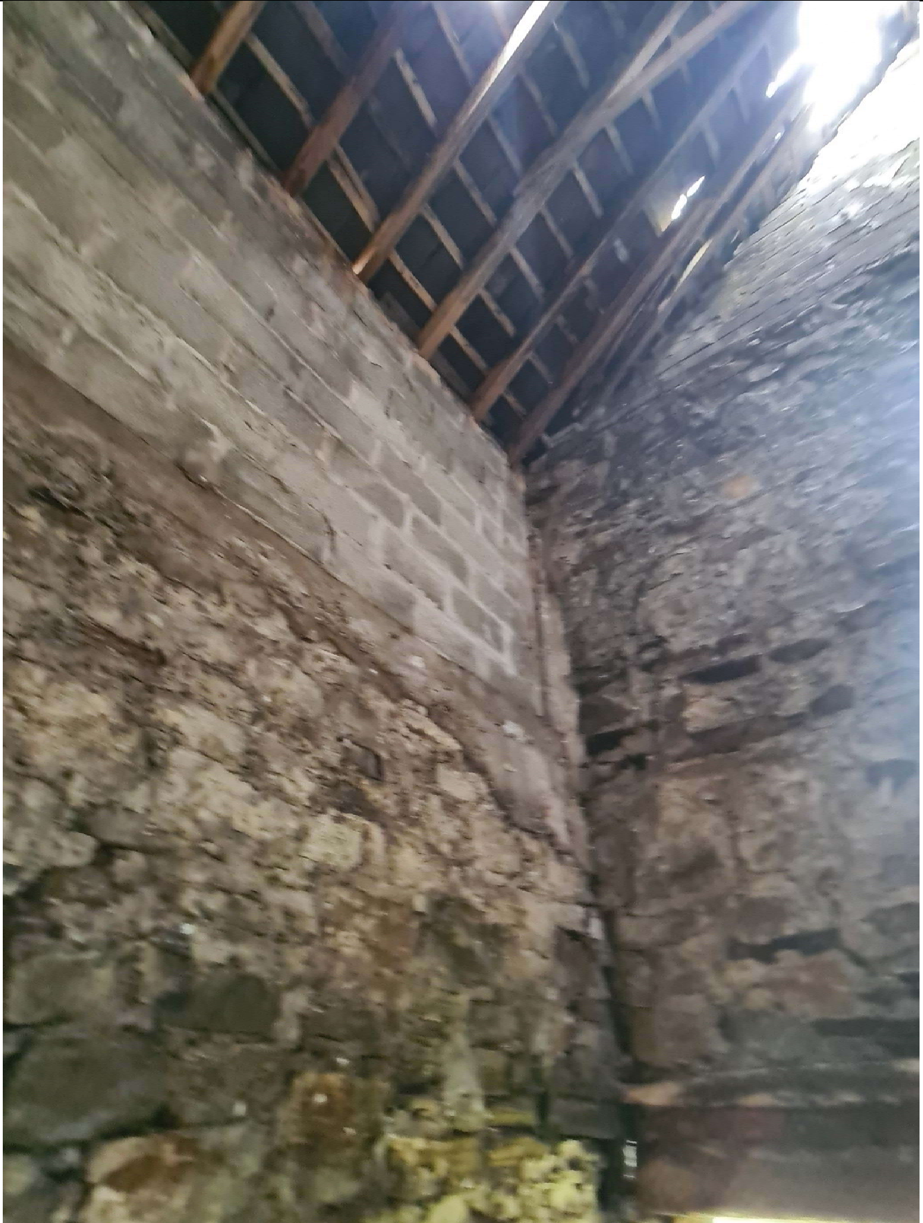
IN19 - Blockwork rebuilt at eaves, suspect due to original failure of roof.
