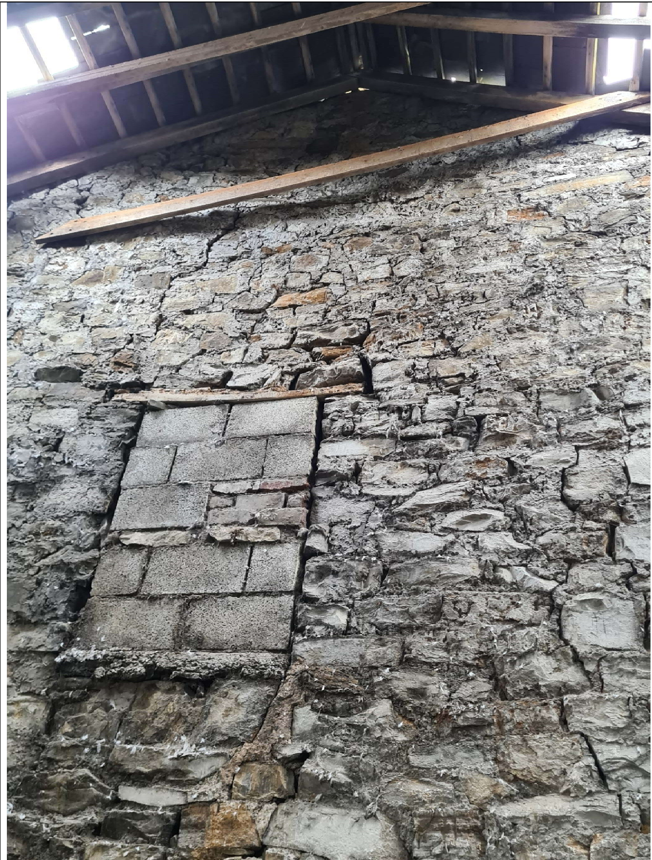
IN21 – Eastern section elevation facing south, failed collar tie at roof, severe cracking and distortion, inappropriate in-fills
