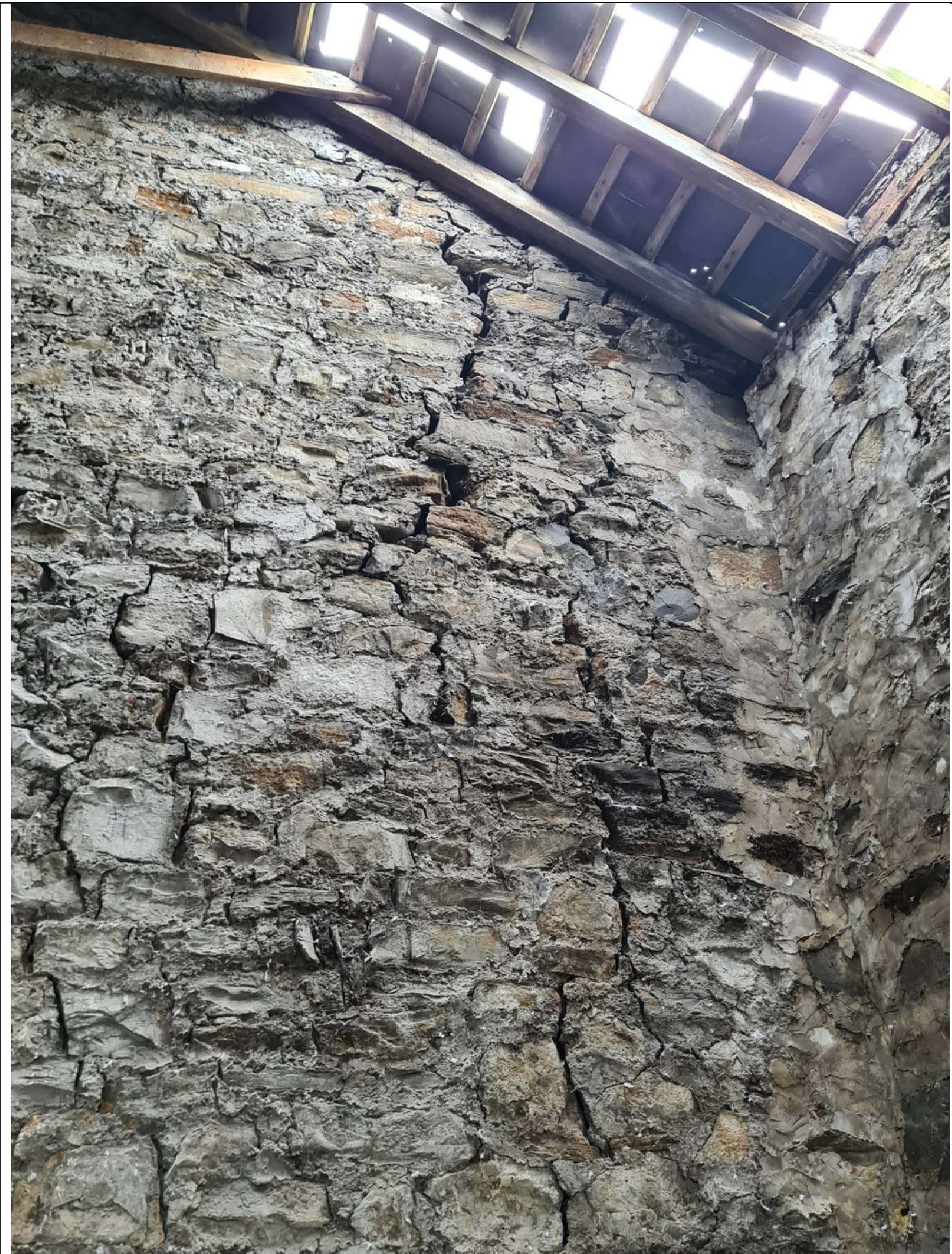
IN20 – Eastern section elevation facing south, severe distortion, vertical cracks and inappropriate repointing
