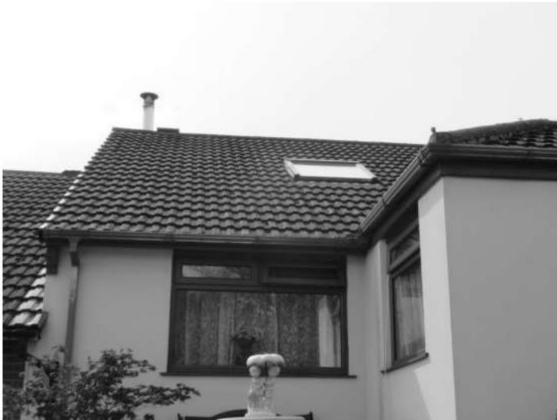
Photograph 3 – The roof and ridge tiles are in excellent condition and are well sealed.
