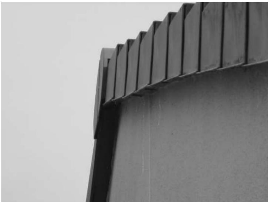
Photograph 10 – The verge capping on the north-western gable end is well fitting with no associated PRFs.
