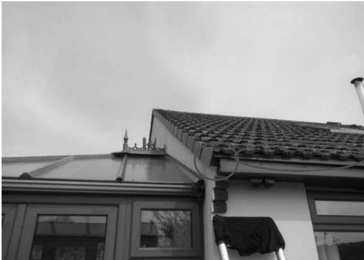
Photograph 7 – Showing the cavities under the end roof tiles and under the roof capping, all of which have temporarily been exposed due to the short-term removal of the guttering.
