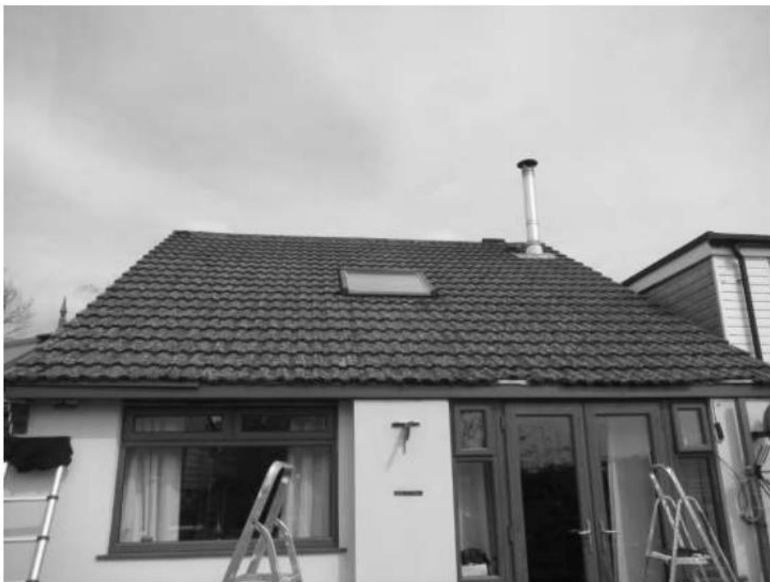
Photograph 6 – Showing the removed guttering and recently painted soffits on the south-western aspect of the building.
