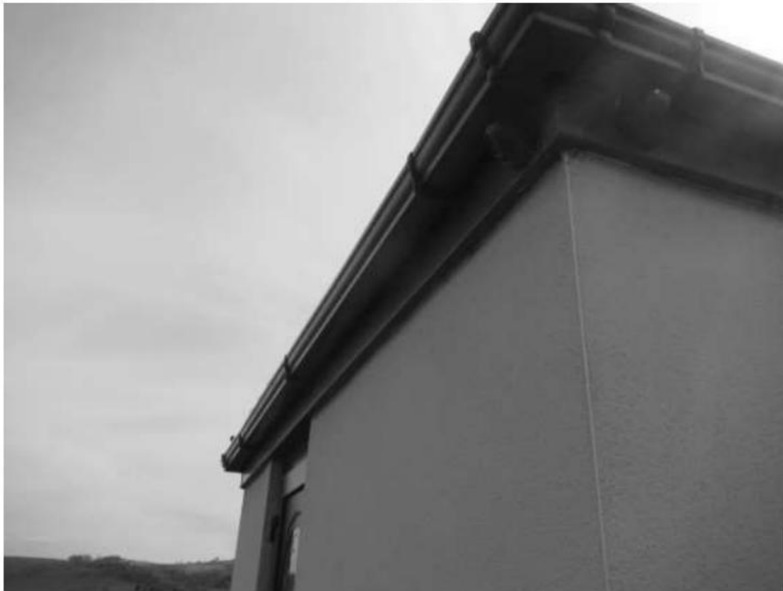
Photograph 5 – The fascias are well fitting with no associated cavities.
