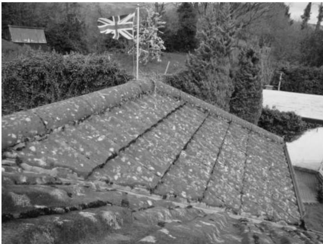
Photograph 4 – The roof and ridge tiles are in excellent condition and are well sealed.
