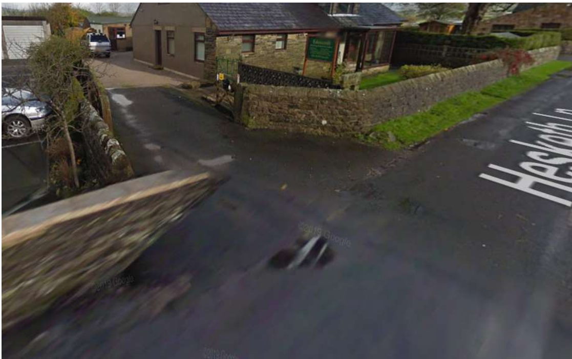
Existing entrance and access from the main road to remain as exists.
