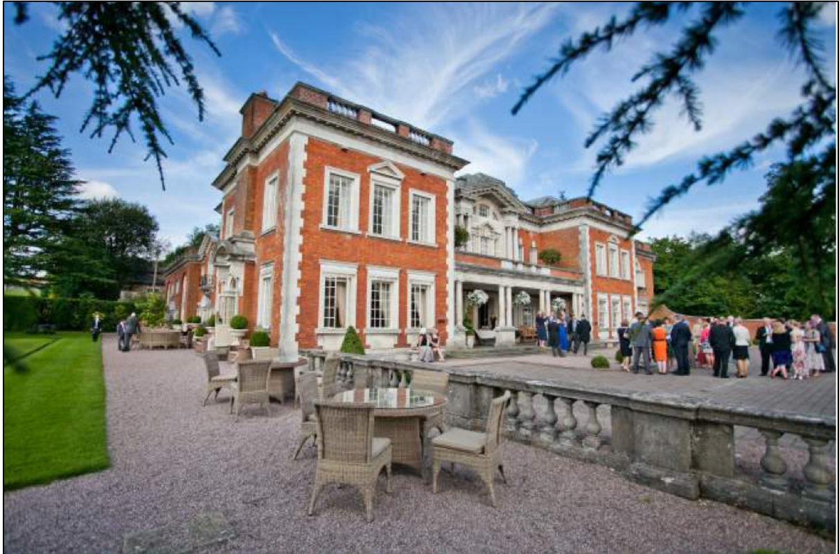
Southern and western elevation of Eaves Hall.
