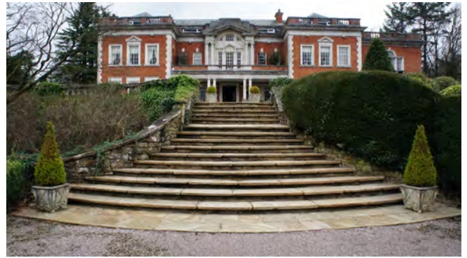
3 View from the south of Eaves Hall frontage
