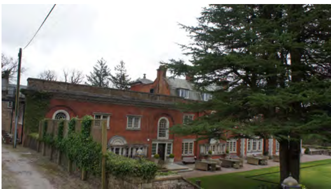
4 View from the northwest of Eaves Hall
