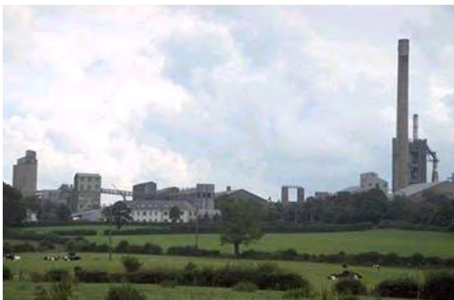
Clitheroe cement works and associated infrastructure
