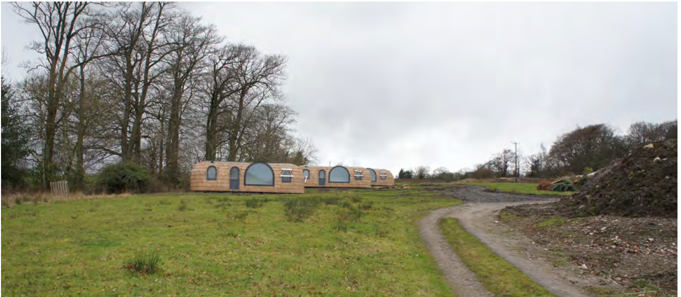
View from southern edge of the site, looking northwest, showing the eco-lodges and access track already constructed
