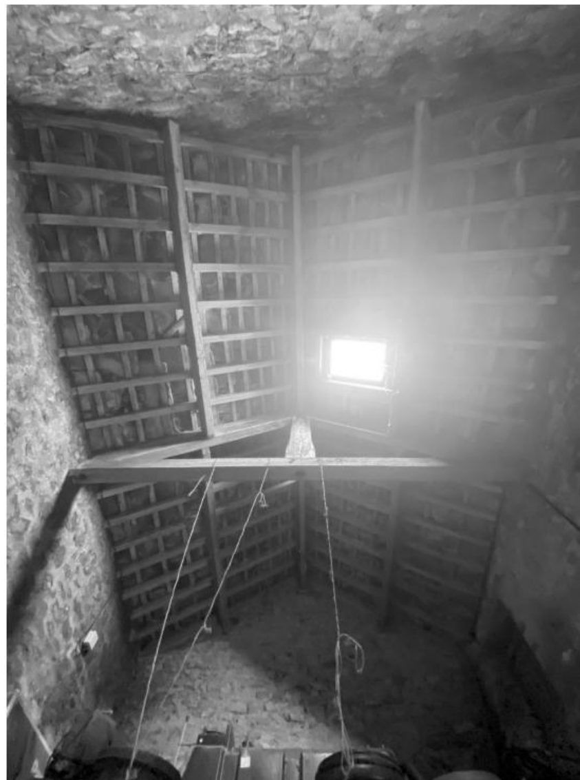
Photo 5: Mistal roof structure
