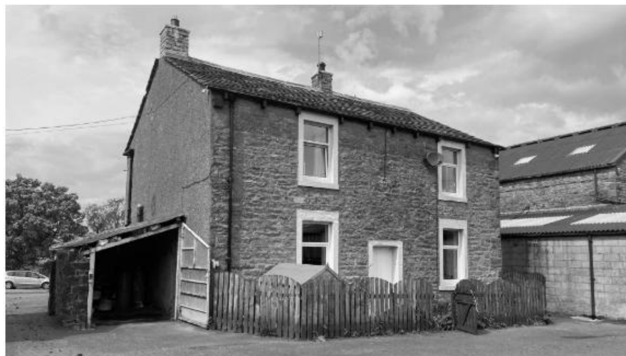
Photo 3: Rear south-east elevation of farmhouse
