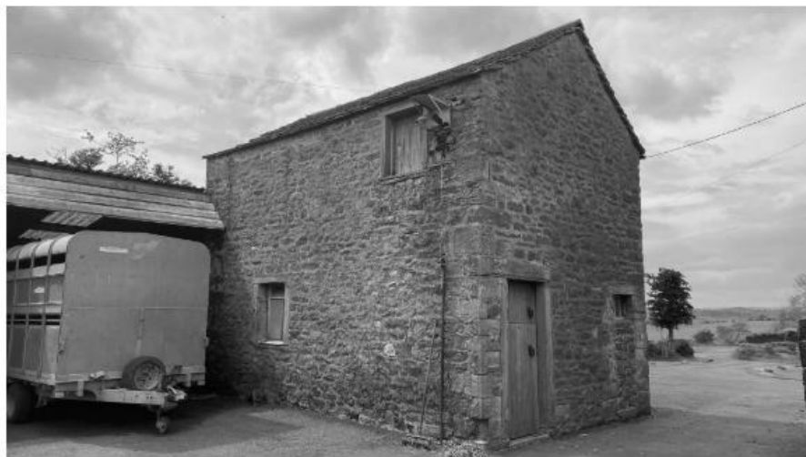
Photo 5: South-east elevation of mistal
