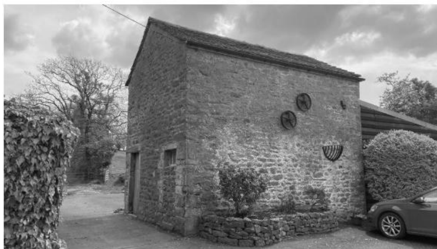
Photo 4: North-west elevation of mistal
