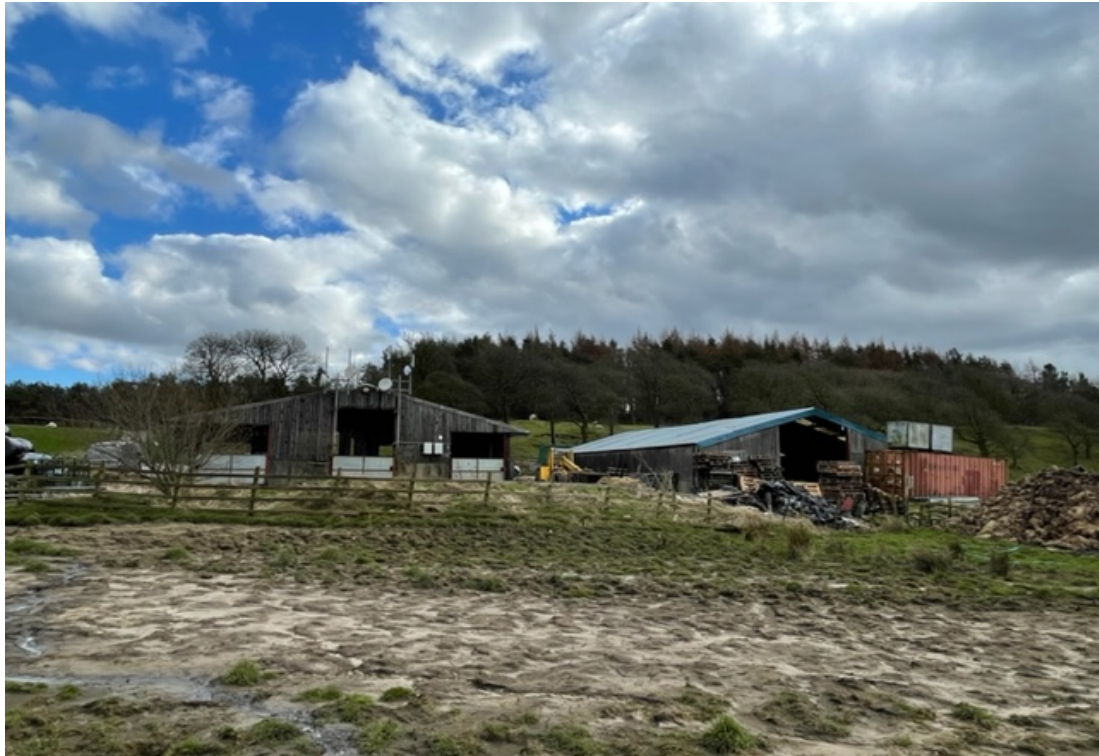
View of the buildings from the north west (plot 1 to the left of the picture)
