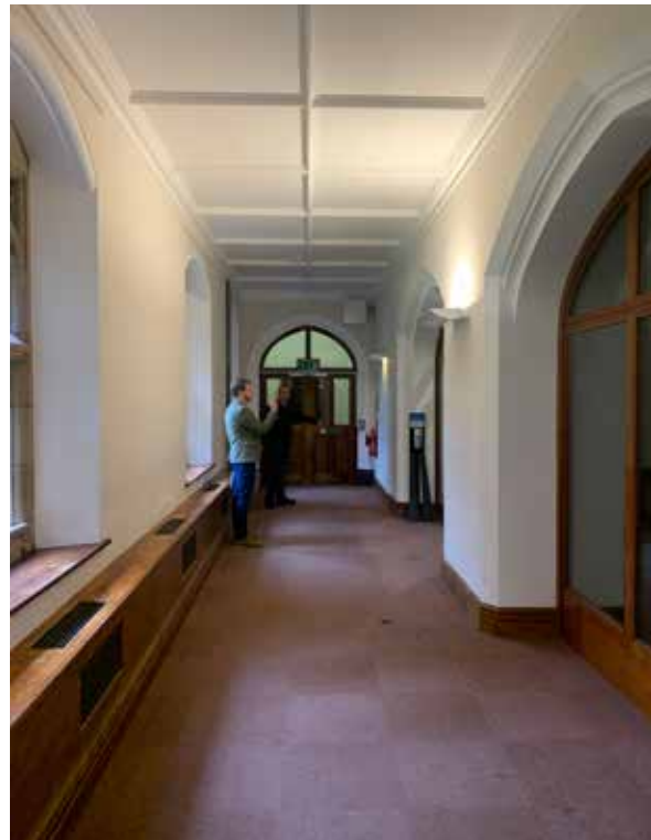
Typical existing corridor with modern arched infills on right
