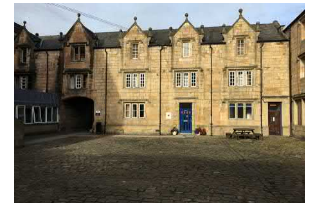
South elevation of North range as it is today
