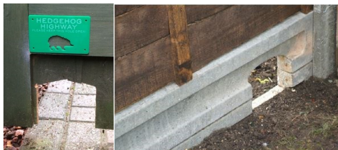
Insert 5: Showing wildlife access gap within fencing
