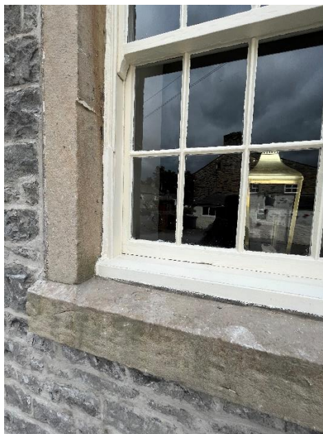
Fig 3 illustrating the seamless repair and repainting of existing window.
