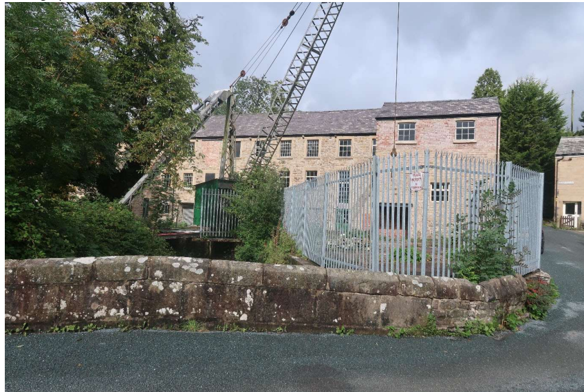
Kirk Mill front bridge
