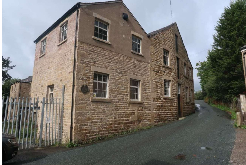
Road elevation Kirk Mill
