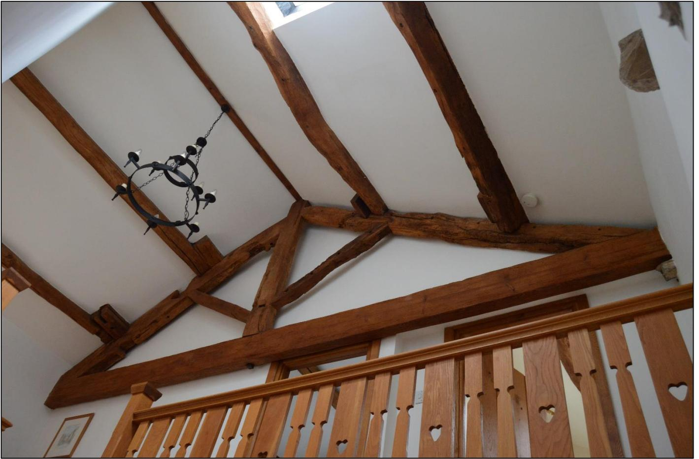
*PLI 6: View of timber kingpost roof truss, purlins and ridge to the first-floor landing.*
