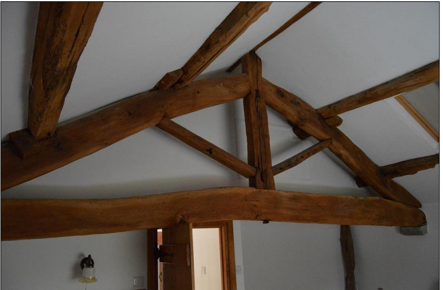
*PLI 7: View of the timber king post roof truss to the first-floor bedroom.*
