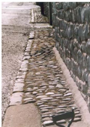
Historic paving in beside No. 1 Ribble Lane
