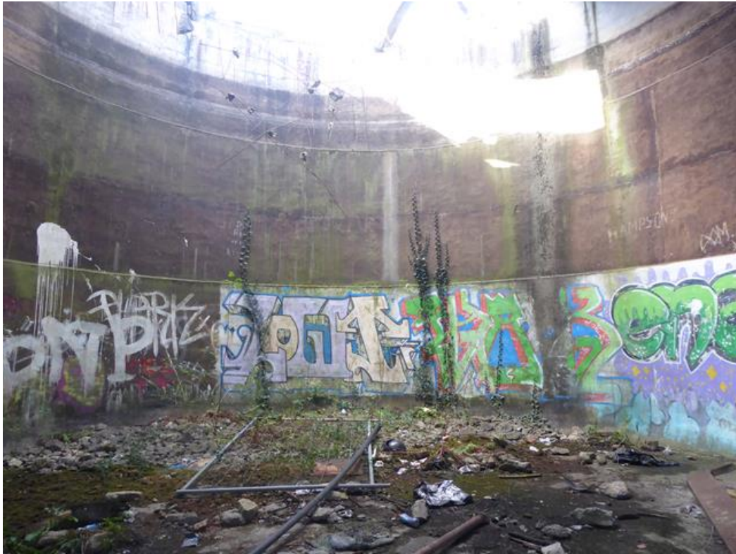
Photo 3: Water Tower interior
