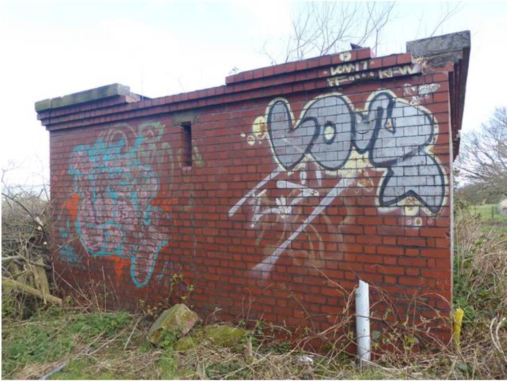
Photo 7: Valve House Southerly Facing Elevation
