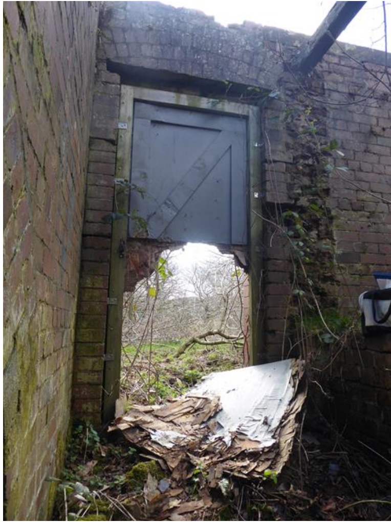
Photo 11: Valve House Door Opening
