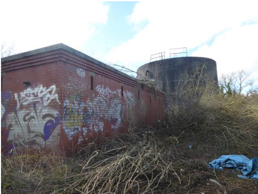
Photo 4: Water Tower and Valve House Northerly Facing Elevation
