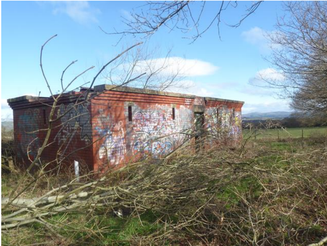
Photo 5: Valve House Southerly Facing Elevation
