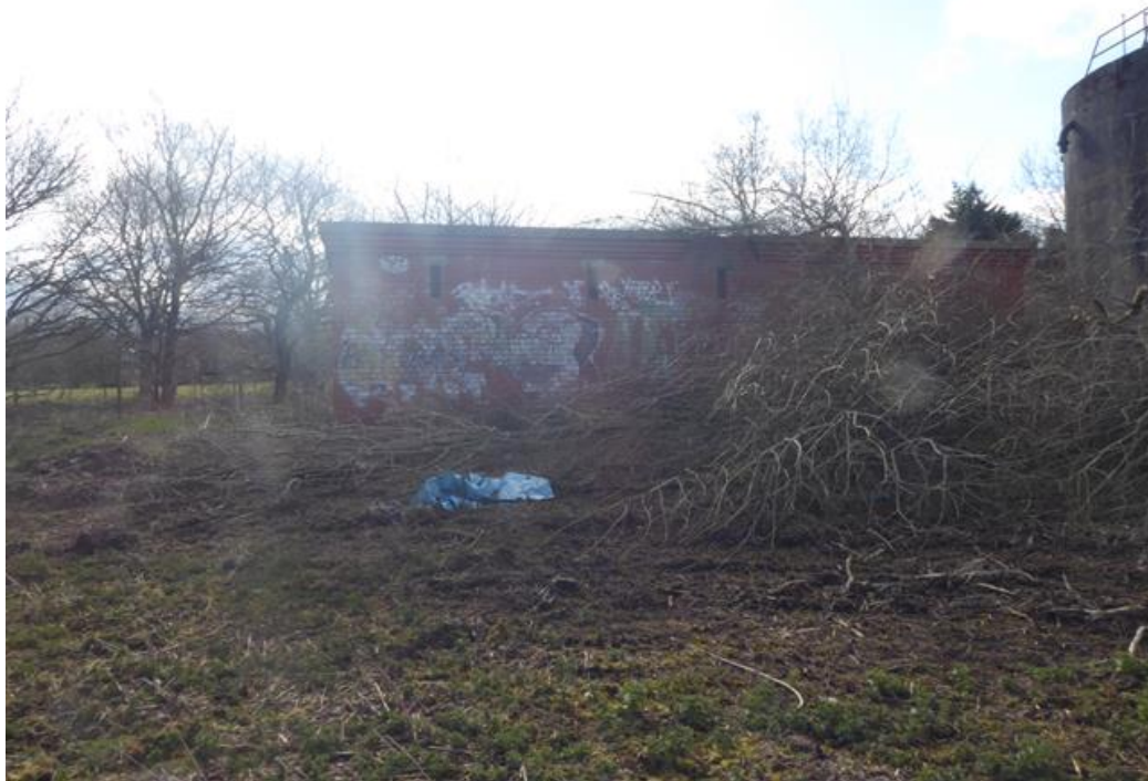
Photo 9: Valve House Westerly Facing Elevation
