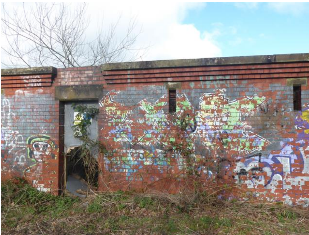
Photo 6: Valve House Easterly Facing Elevation
