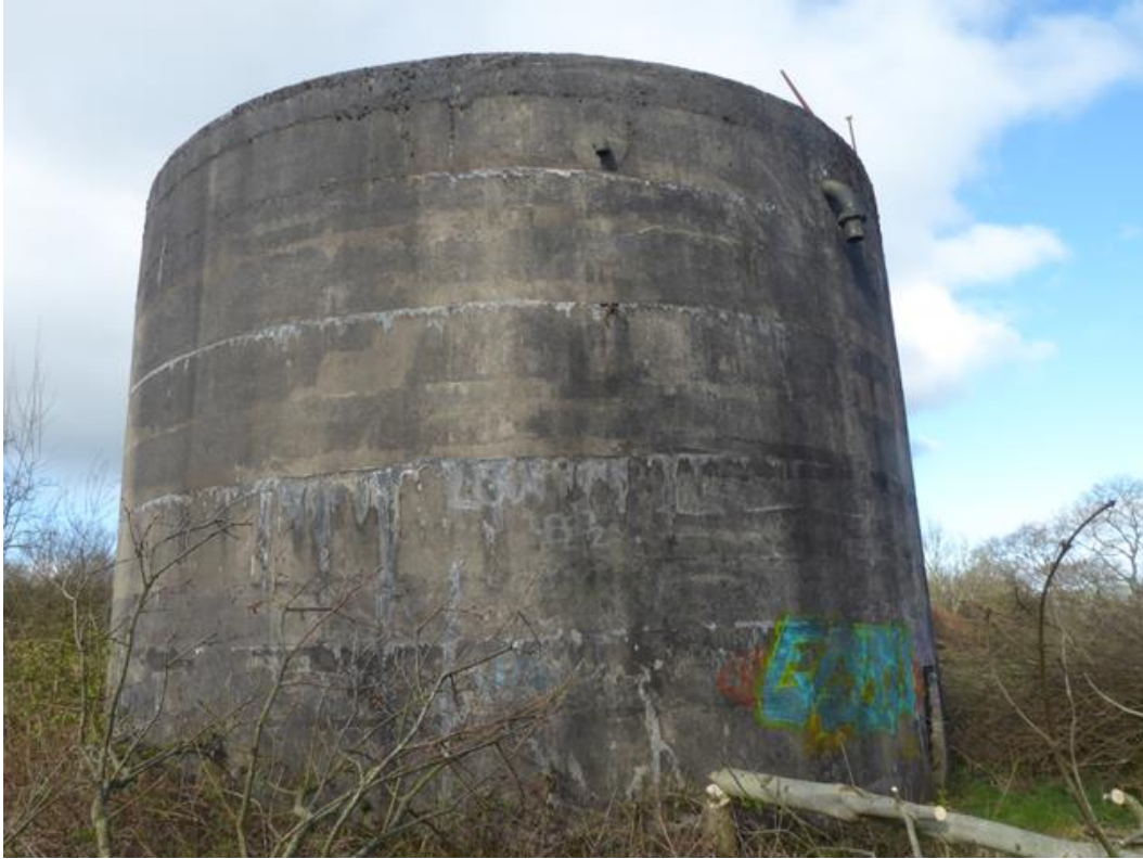
Photo 1: Water Tower Easterly Facing Elevation
