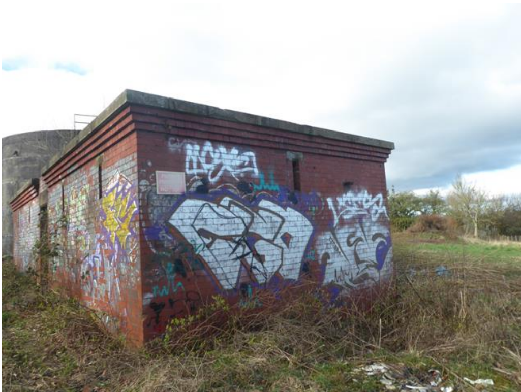
Photo 8: Valve House Northerly Facing Elevation
