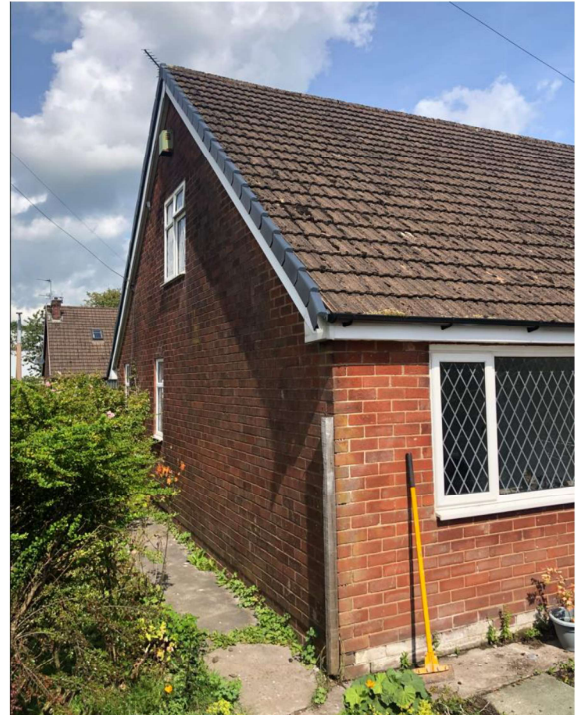
Photograph 3: View of the side (south) elevation which shows the plastic soffits and concrete roof in good condition and no gaps present.
