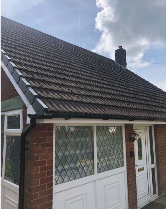
Photograph 1: View of the front (west) elevation of the property. Brick wall and concrete tile roof.
