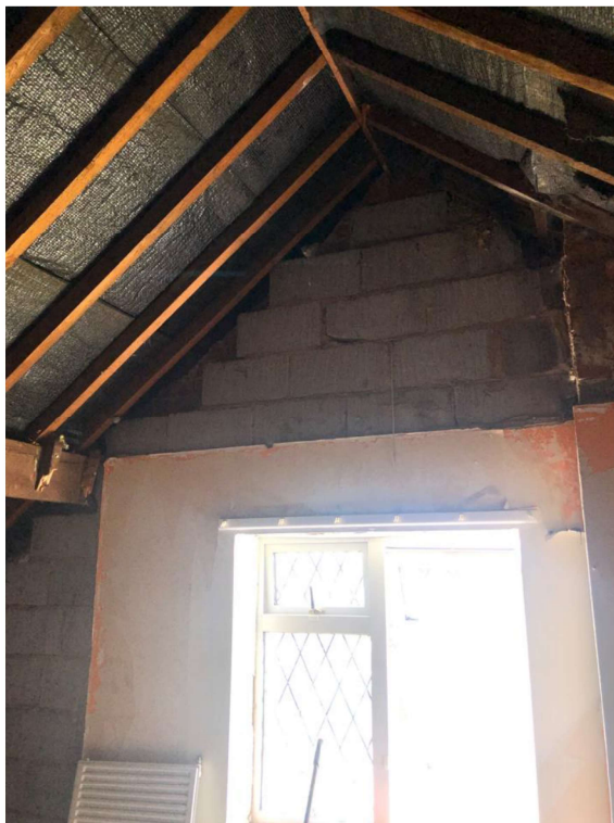
Photograph 5: Internal roof space used as bedroom. Internal walls knocked down and exposed roof. Concrete tiles underlay with geotextile material.
