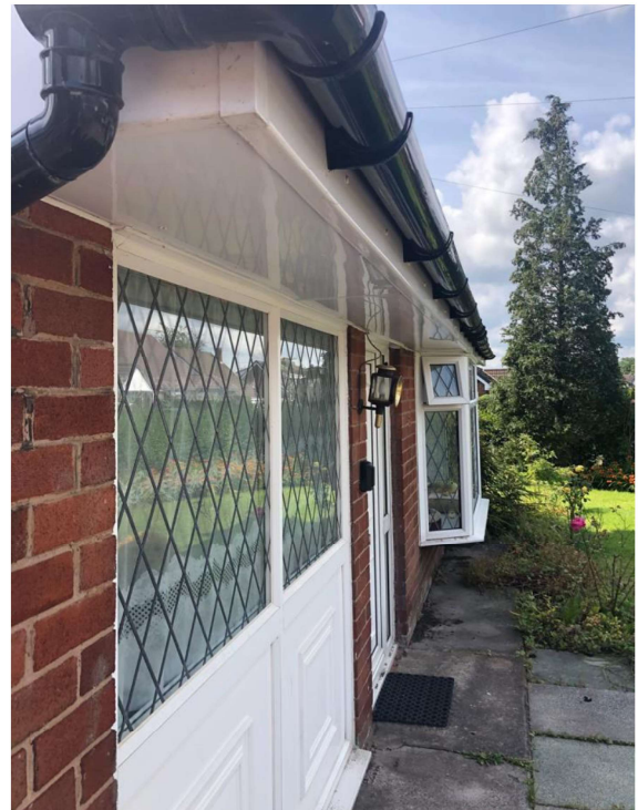
Photograph 4: Close up of the plastic soffits which were all installed approximately two years ago.
