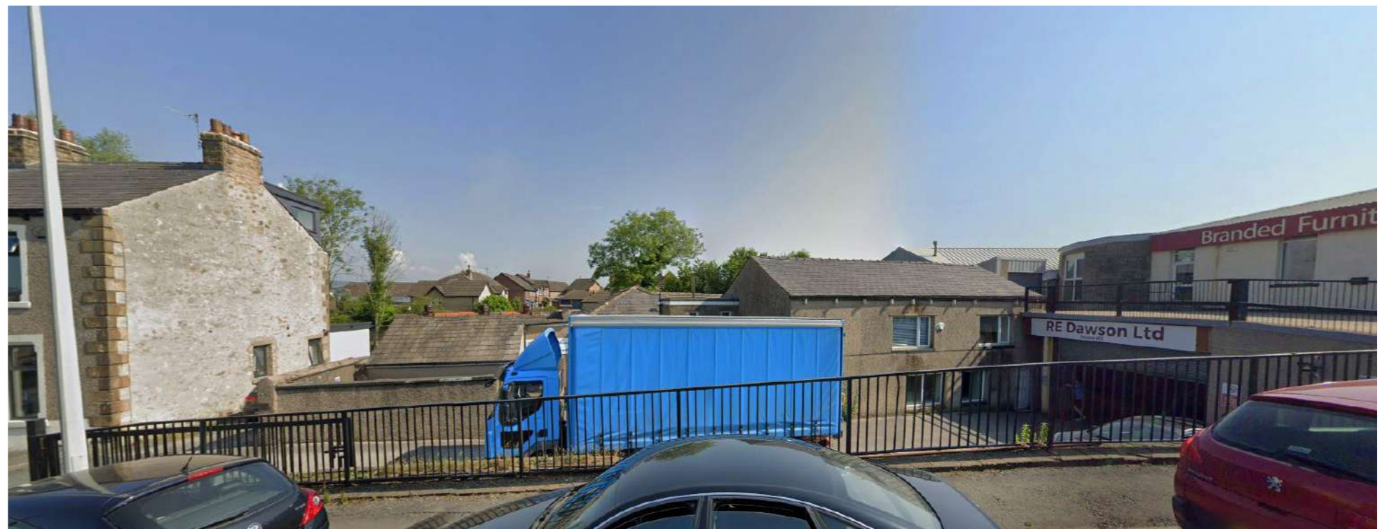
Approach Four - South west boundary showing loading area and courtyard.
