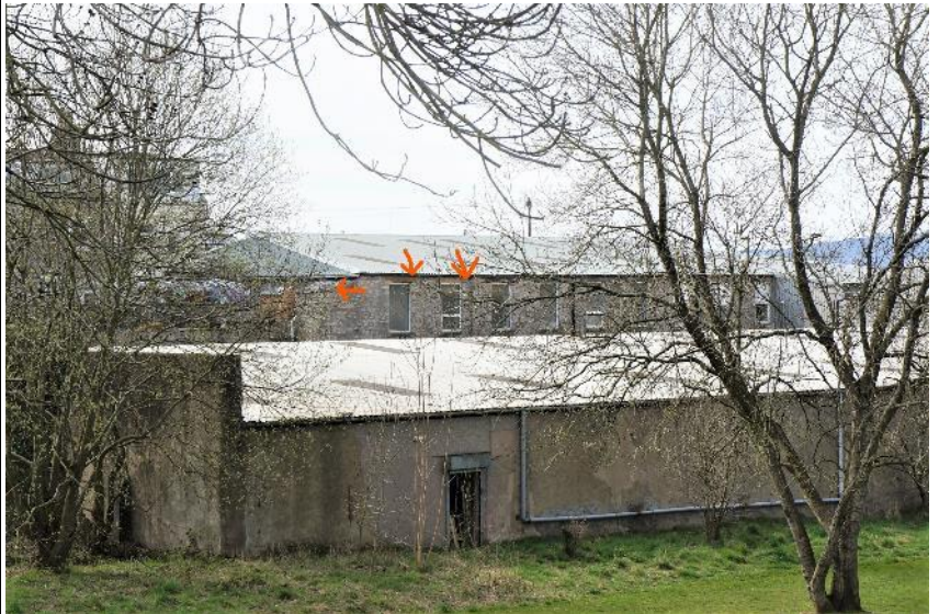
Figure 19: B2 East elevation showing small outbuilding, and north elevation with gaps in window lintels on the upper storey.
