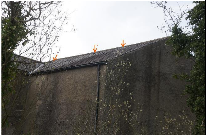
Figure 23: B3 Eastern roof pitch of western-most section , with gaps in roofing materials marked in red.
