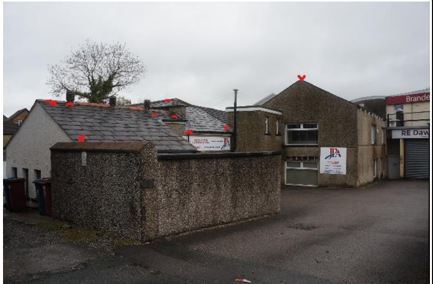
Figure 20: B3 west and south elevations, with gaps in roofing materials marked in red.
