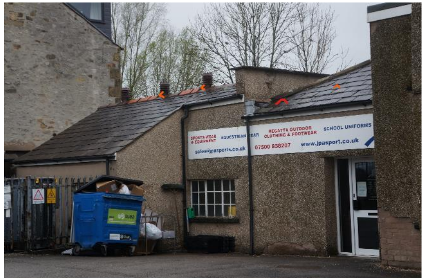
Figure 21: B3 west and south elevations, with gaps in roofing materials marked in red.
