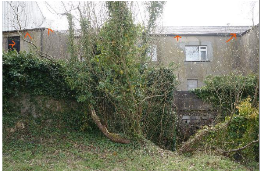
Figure 24: B3 North elevation , with gaps in roofing materials marked in red.
