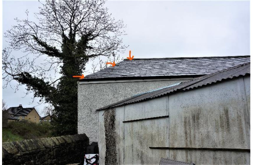
Figure 22: B3 far west elevation, with gaps in roofing materials marked in red.
