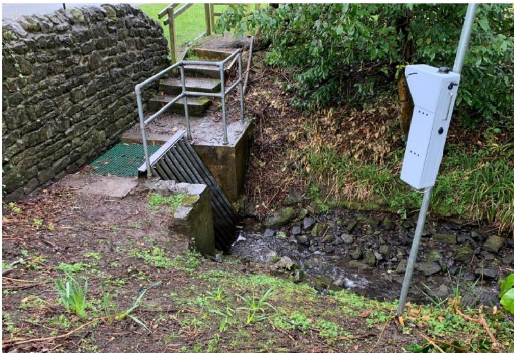
Figure 4: Shaw Brook Upstream Culvert Headwall
