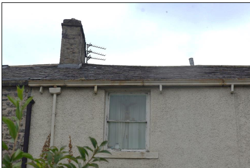
Photo 3: Rear elevation of the main roof. Some tiles have lifted leaving large gaps behind.
