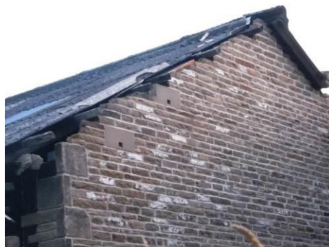
Example of Forticrete boxes in situ
