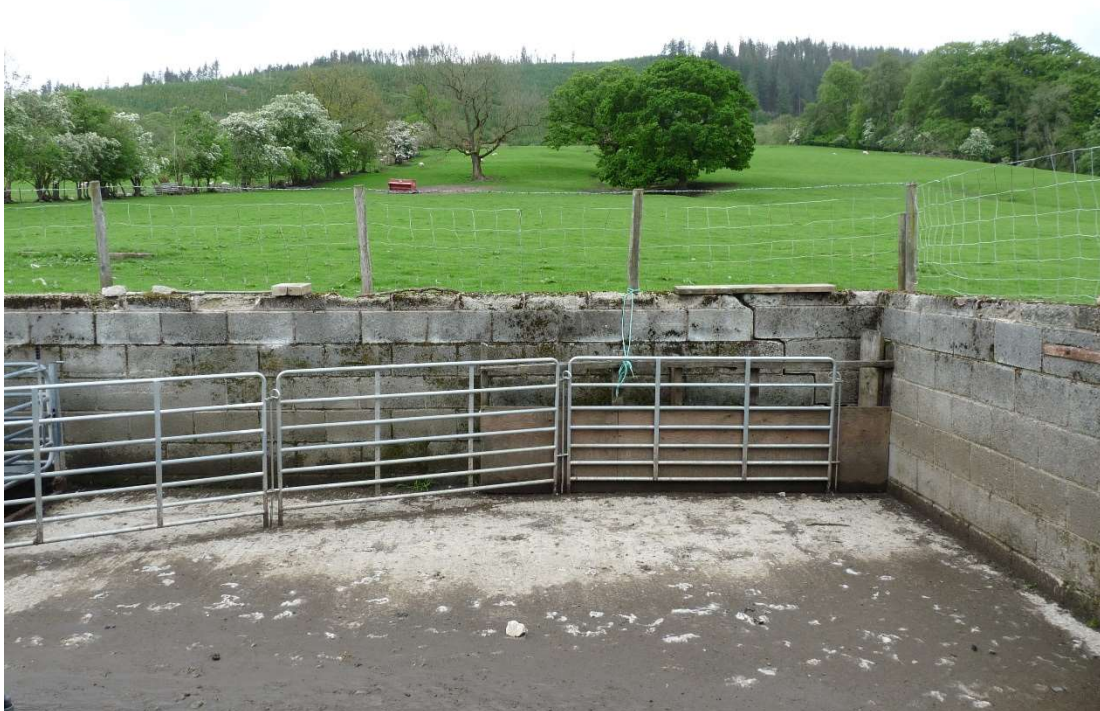
View from proposed patio uphill wall rebuilt with stonework
