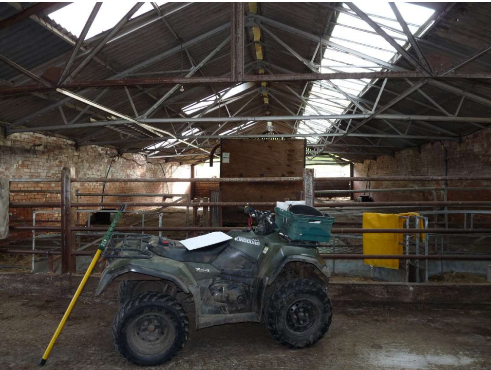
Internal structure quad storage not secure
