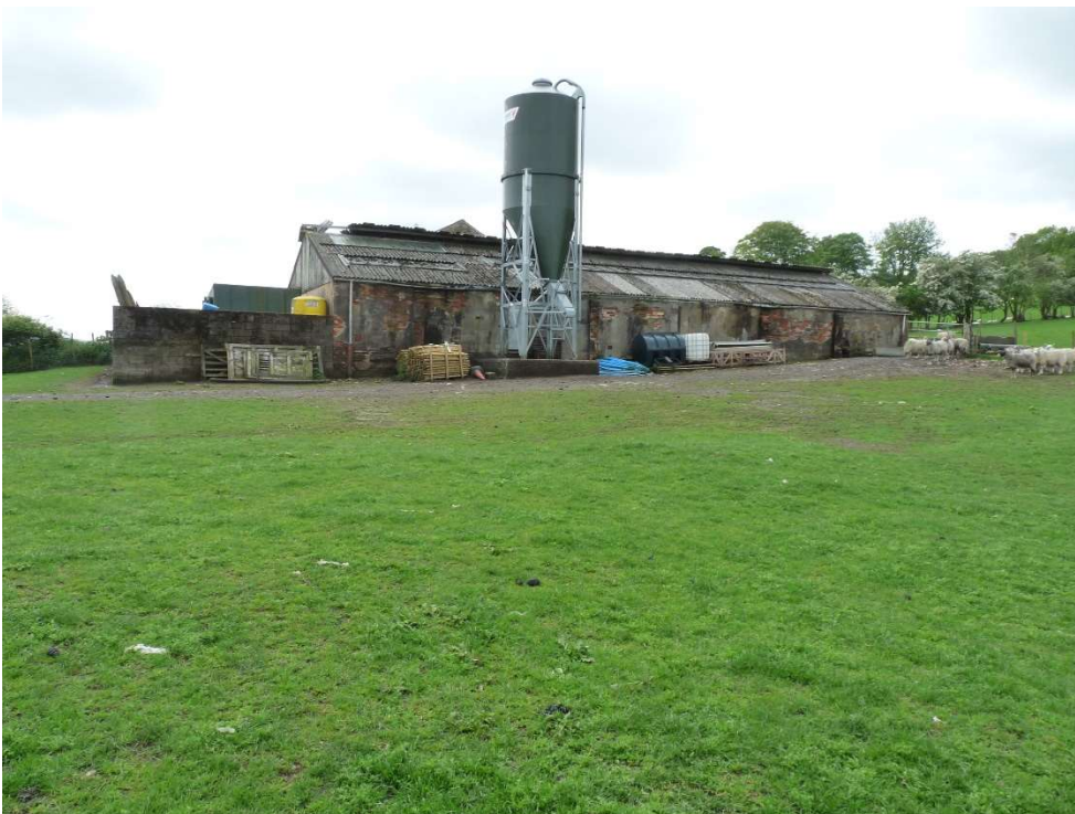
Elevation to field silo, portacabin, lorry and wall removed
