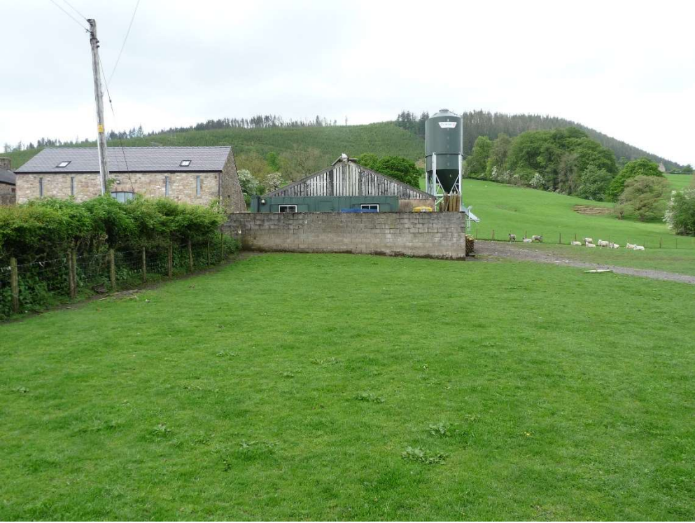
Front from field silo,office,loo removed wall changed to stone
