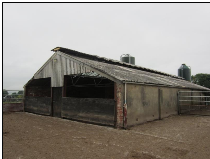
Photo 2: East gable and south elevation of the shippon
