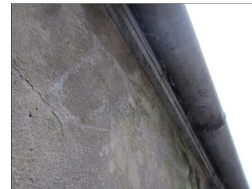
Photo 2: Tightly sealed timber fascia at shippon; no opportunities for roosting bats
