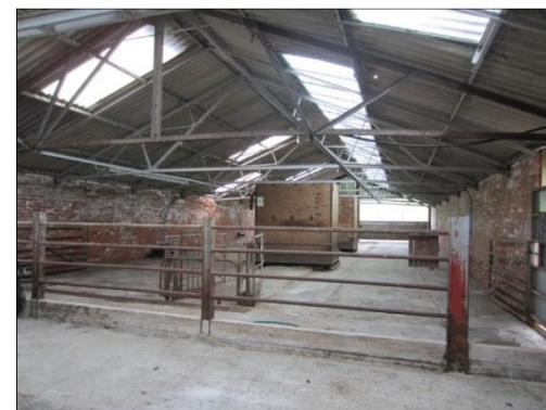
Photo 3: Interior of the shippon (facing west). Mortared internal brick walls; no gaps for bat access.
