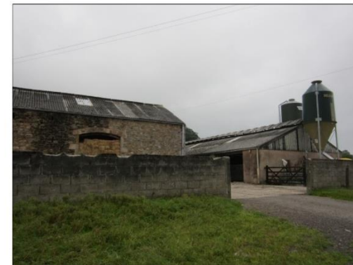
Photo 1: Shippon (right) and adjacent stone barn (left)
