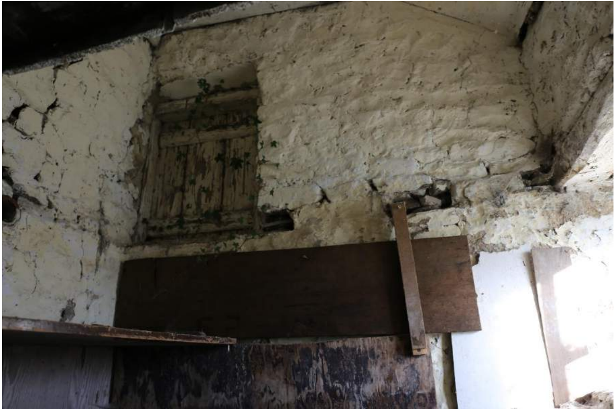
Plate 30: Hatch into upper part of outbuilding, facing north-east
