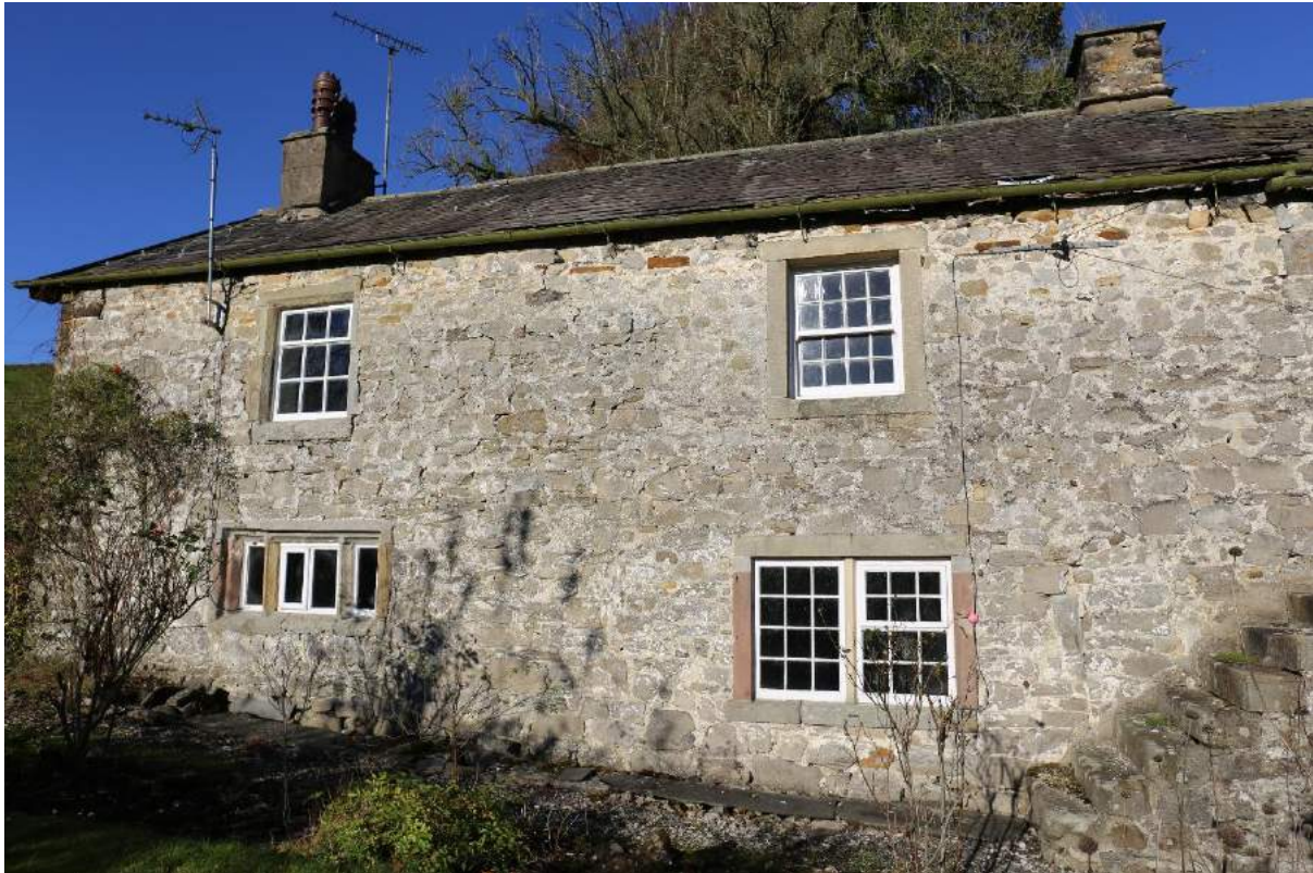
Plate 21: Four-pane mullion window and sash windows to rear of farmhouse.
