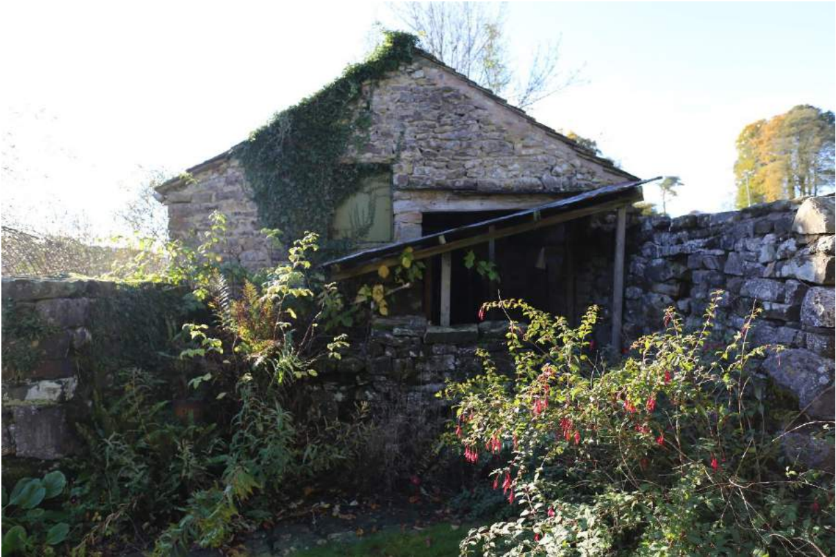
Plate 26: Outbuilding, facing south-west
