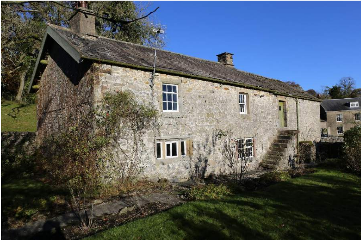
Plate 9: Knott Gate, facing north, showing the farmhouse, the adjoining cart shed outbuilding and steps up (right of frame).
