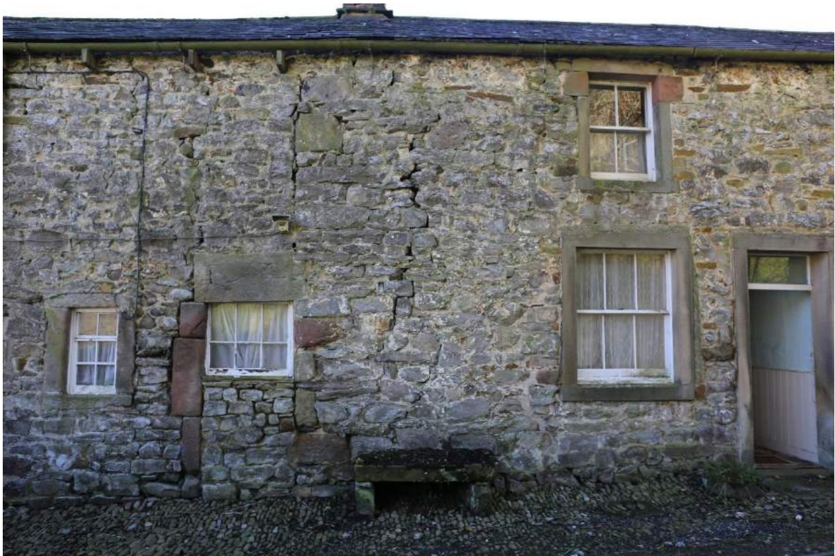
Plate 31: Ground floor window that replaces a blocked doorway, with discoloured sandstone quoins. Note the cobbled flooring and stone bench.
