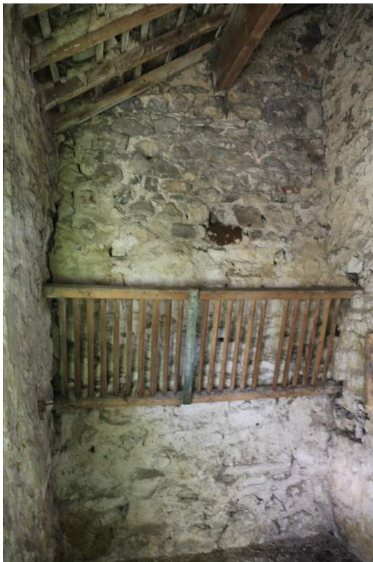
Plate 28: Feeding stall in outbuilding, facing south-west
