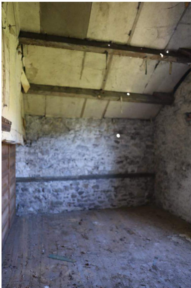
Plate 16: First floor, bare room above garage
