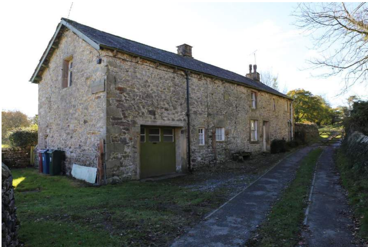
Plate 19: Full range, general view facing south
