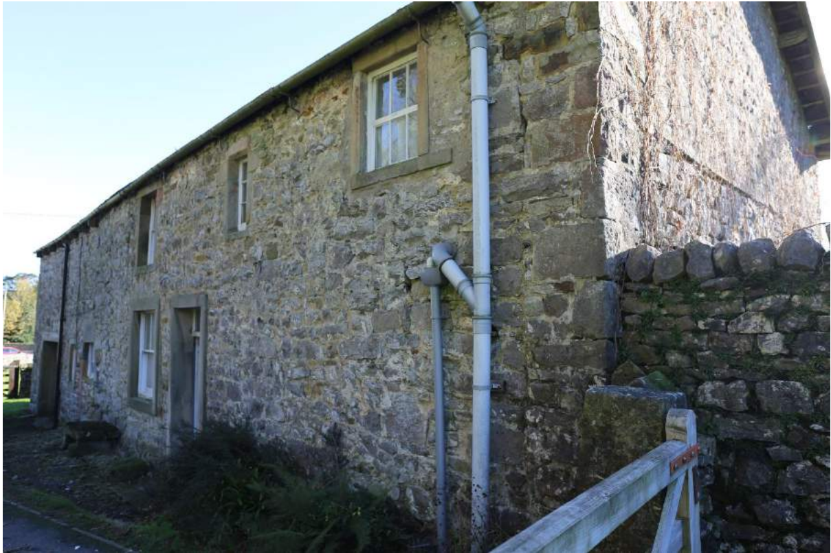
Plate 24: Oblique general view of the front elevation, facing east-north-east
