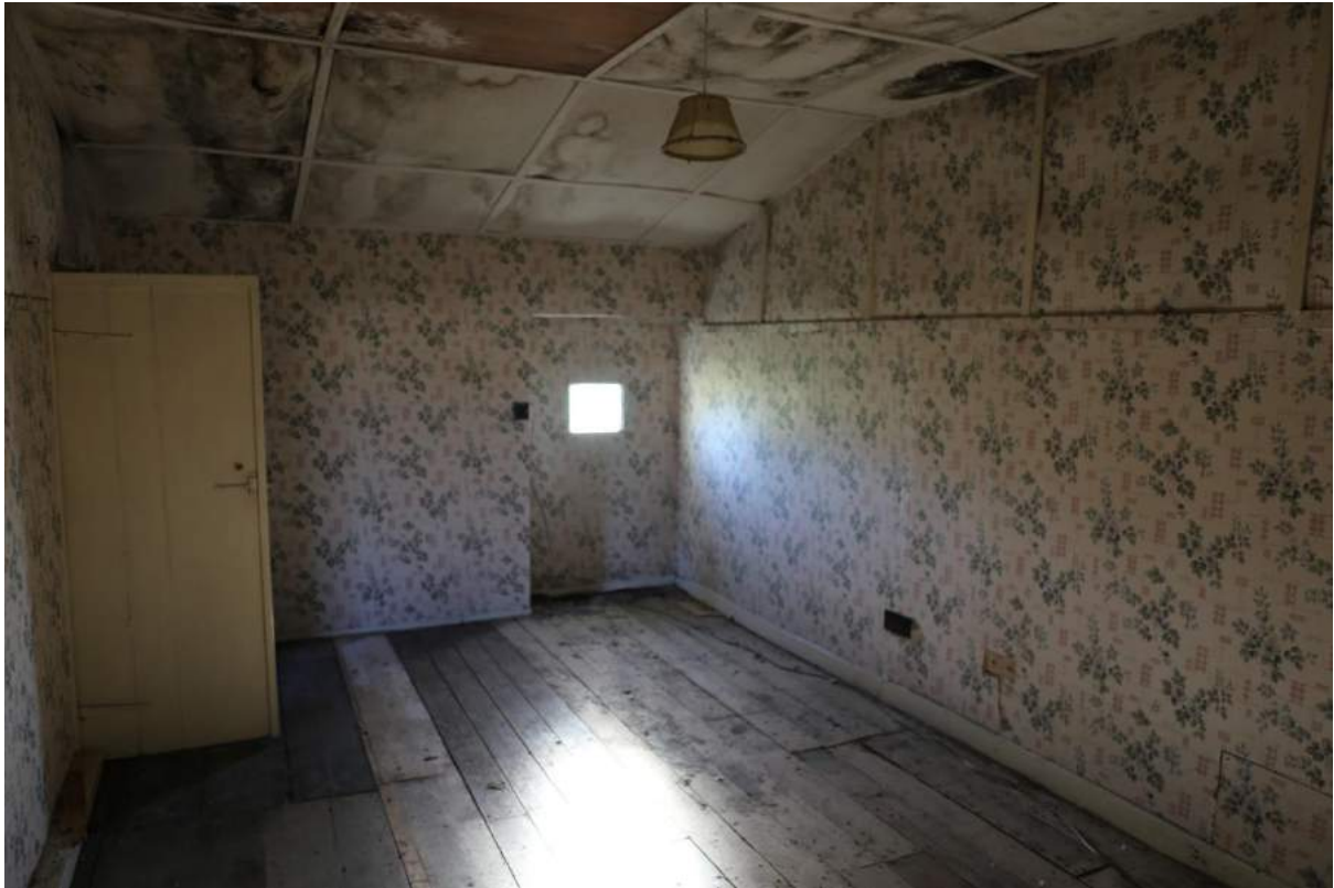
Plate 17: First floor, bedroom in upper floor over kitchen, note blocked doorway
