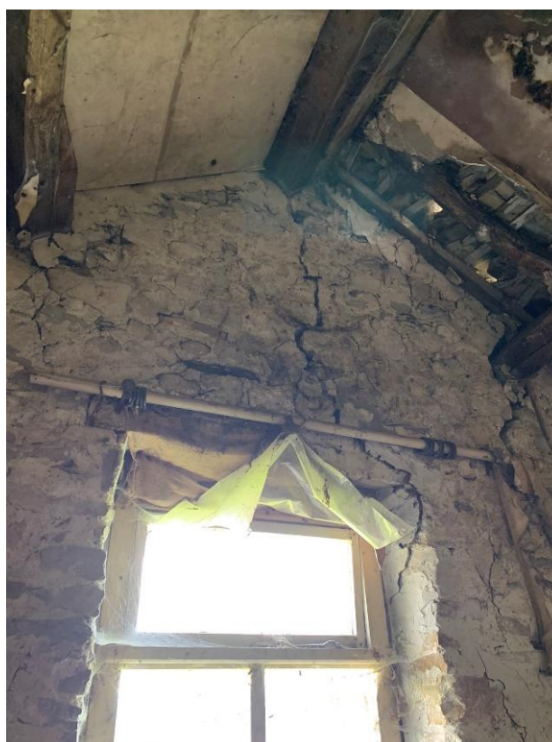
Internal Gable Wall
