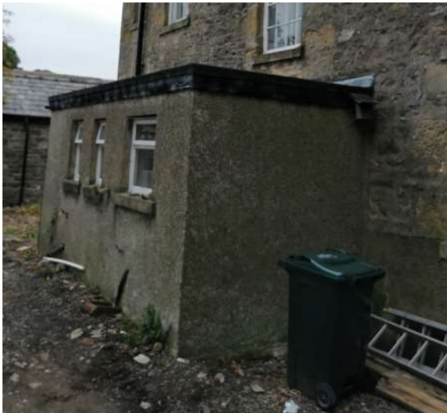
FIGURE 4: IMAGE OF THE EXISTING FLAT ROOF REAR STRUCTURE TO BE REMOVED
