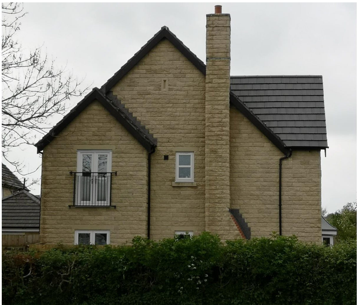
A view of the gable (east) elevation.
