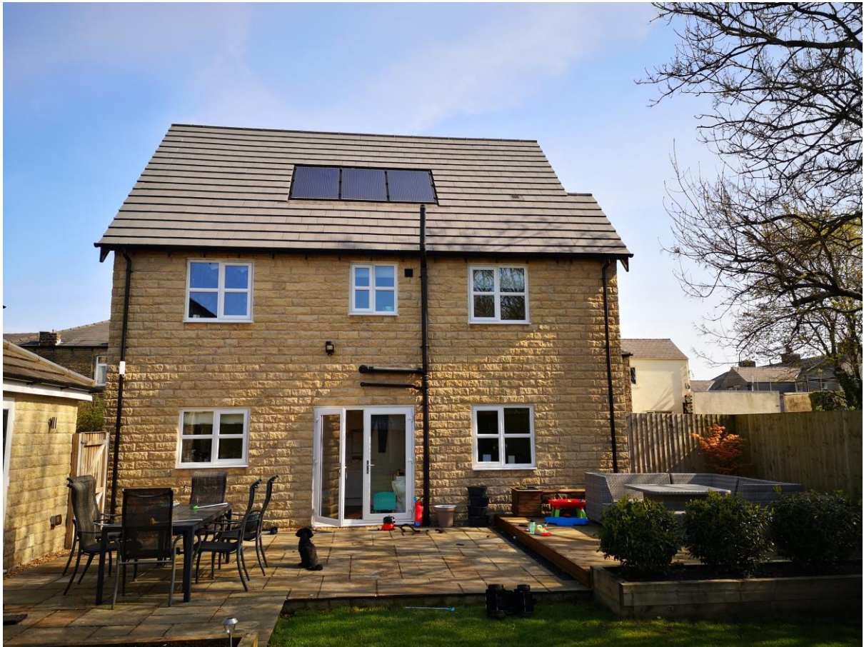
A view of the rear (south) elevation where the proposed extension will be sited.
