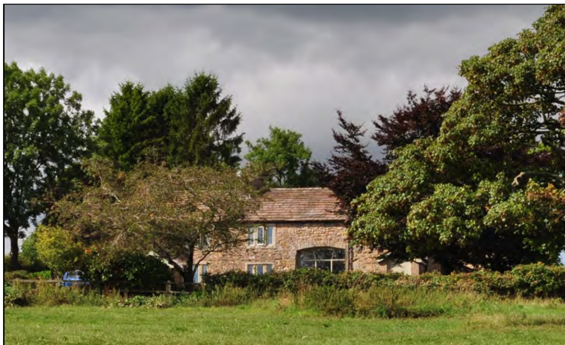
Photo 3: Eaves House Cottage and barn
