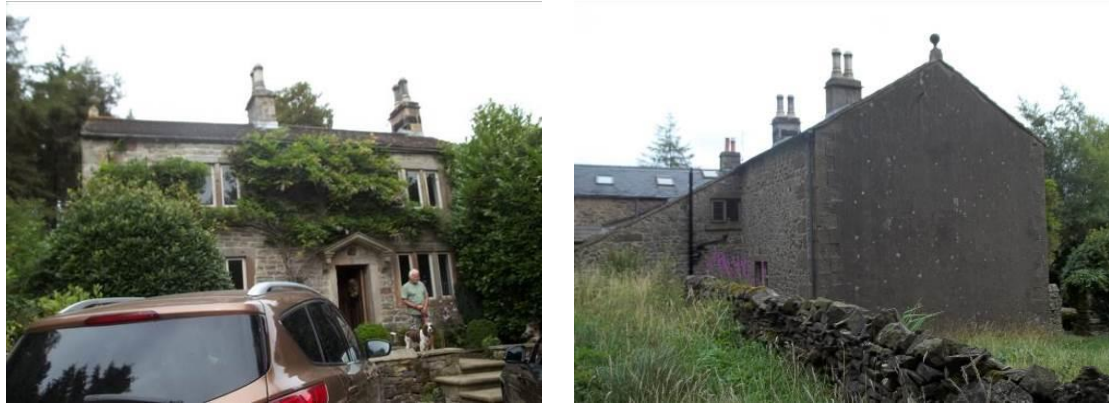
Front (south-east) and south-west-side/rear elevations
