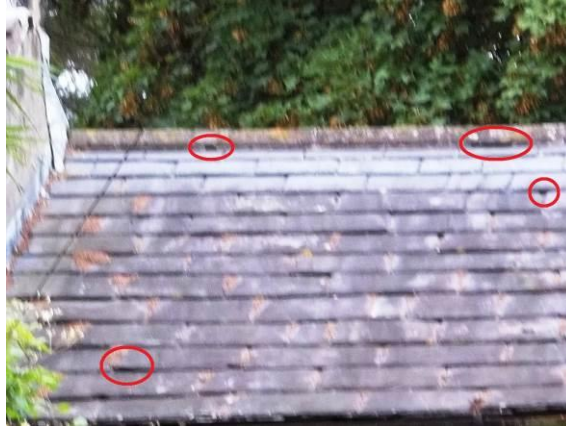
Plate 15. Examples of potential bat access gaps illustrated in red
