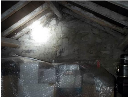
Plate 3. South-west and north-east gable ends
