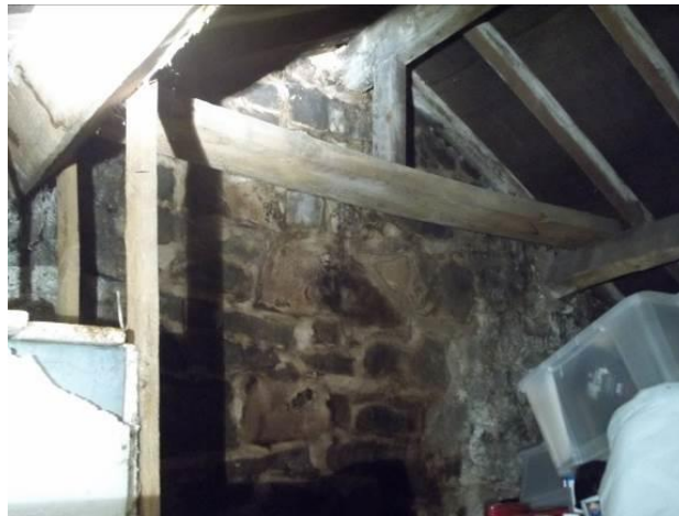
Plate 1. North-east gable end
