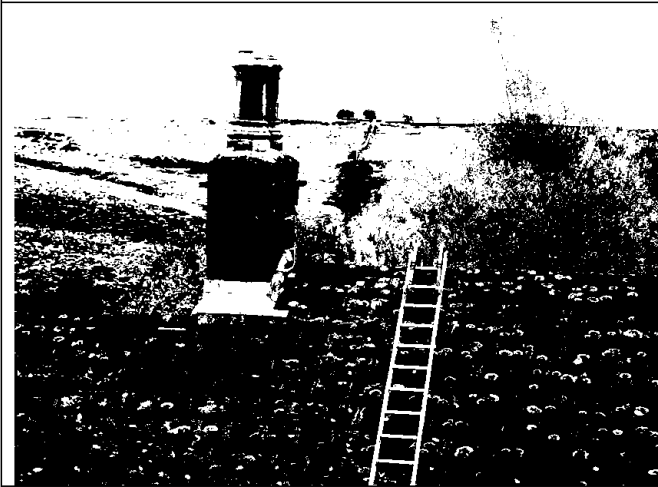
Photo 7 – Rear elevation of roof / chimney
