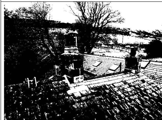
Photo 3 – Chimney to front elevation .
