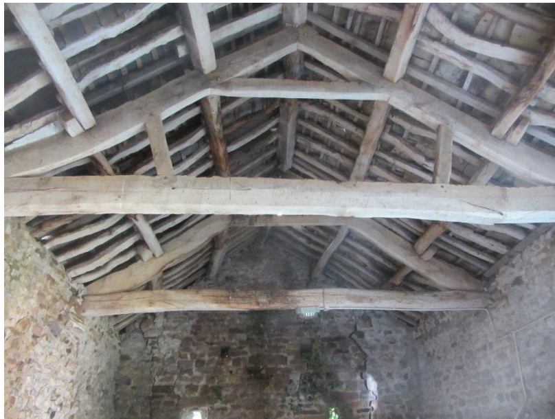
Photo 3 – Internal view of northern space looking north
