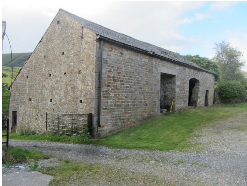
Photo 1 - View of building from south east
