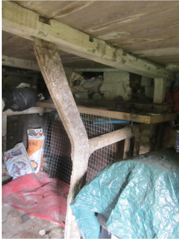
Photo 9 – Internal view of timber structure supporting loft floor
