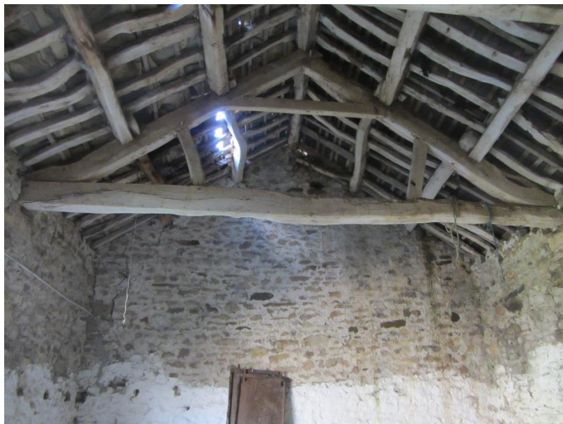
Photo 4 – Internal view of northern space looking south
