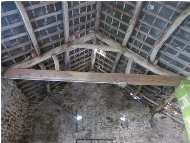
Photo 6 – Internal view of southern space looking south
